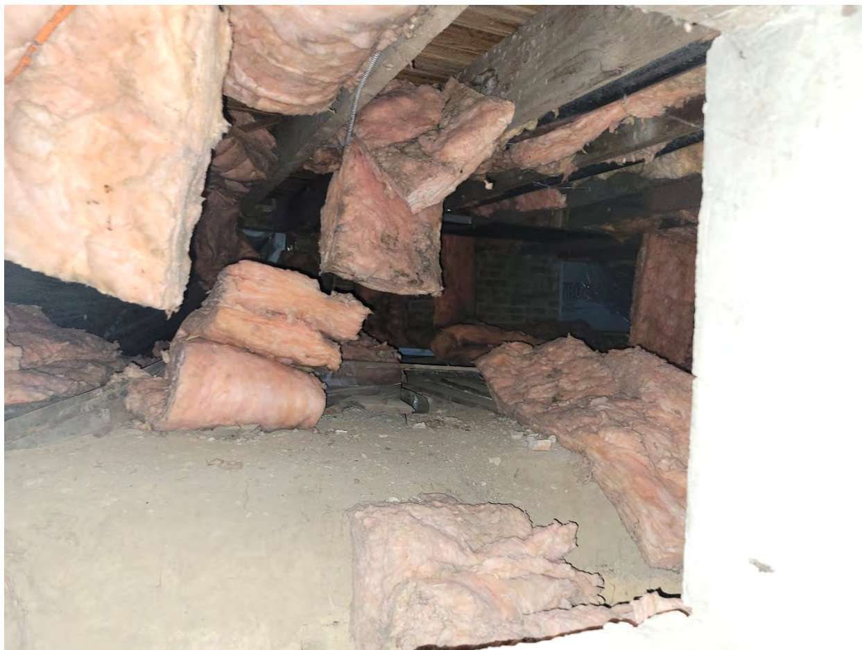
Image 2.3.11: Crawl space under the front third of the greenskeeper's house.
