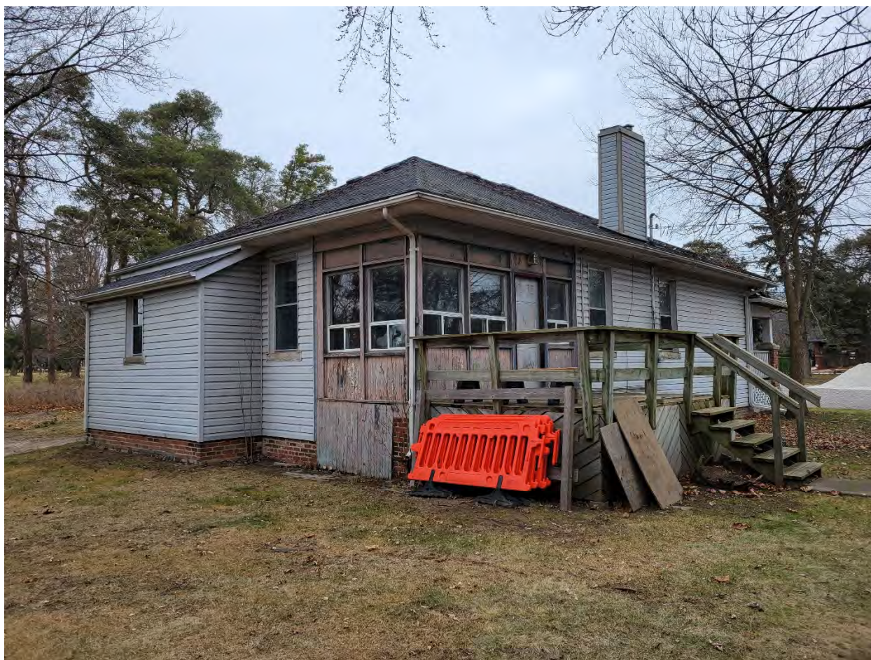
Image 2.3.8: South corner of the greenskeeper's house. Source: +VG Architects.
