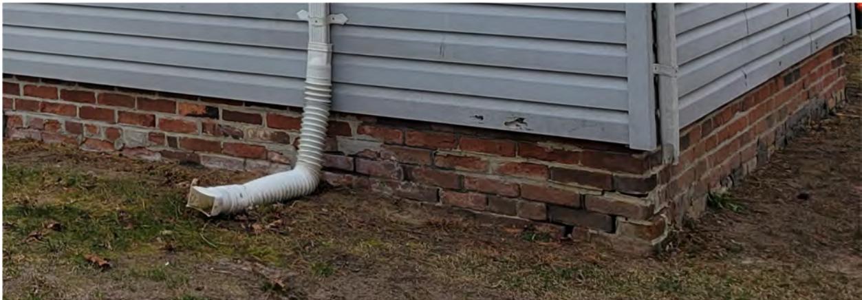
Image 2.3.9 and 2.3.10: Brick foundations at the north side. Source: +VG Architects.
