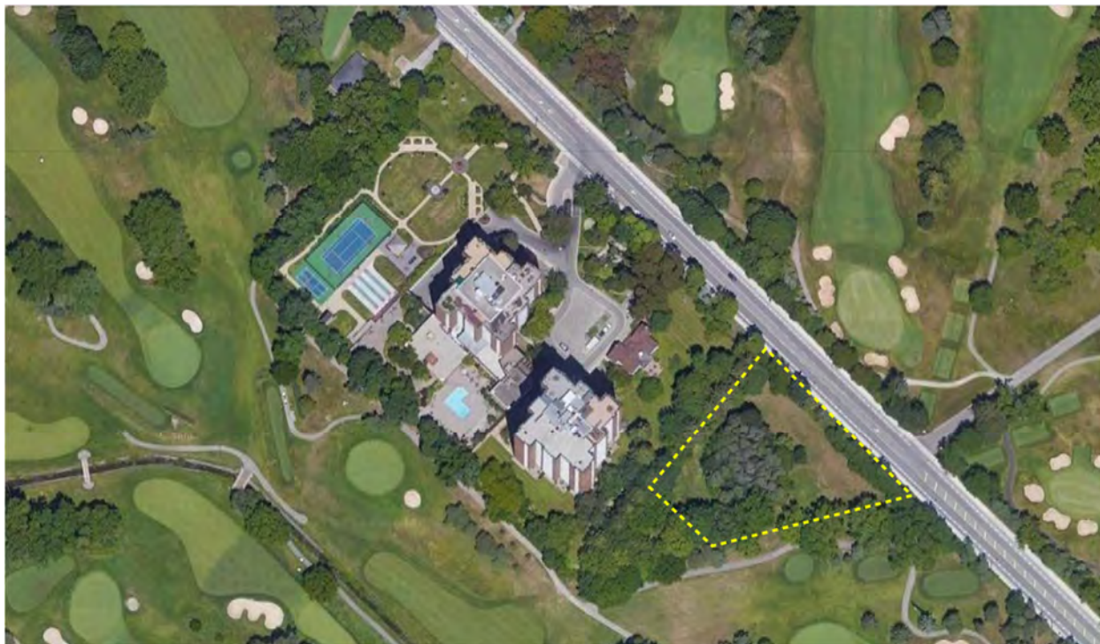
Image 2.6.1: Aerial view of the proposed site for Option 3. The approximate boundary of the site is shown with a yellow dashed line.
