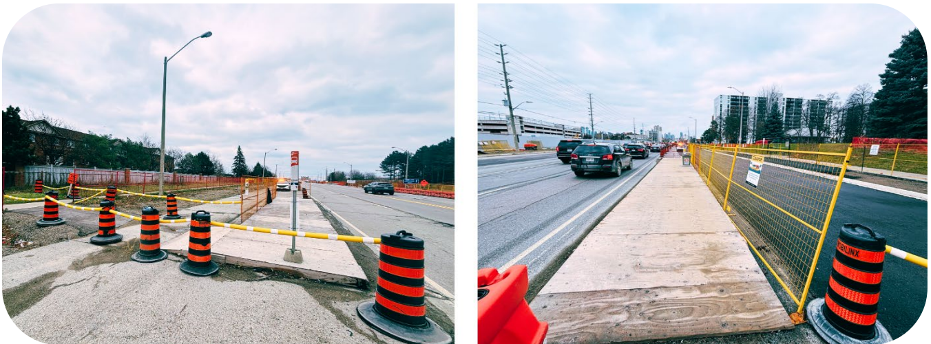
Figure 7: Temporary pedestrian walkways and ramps.
