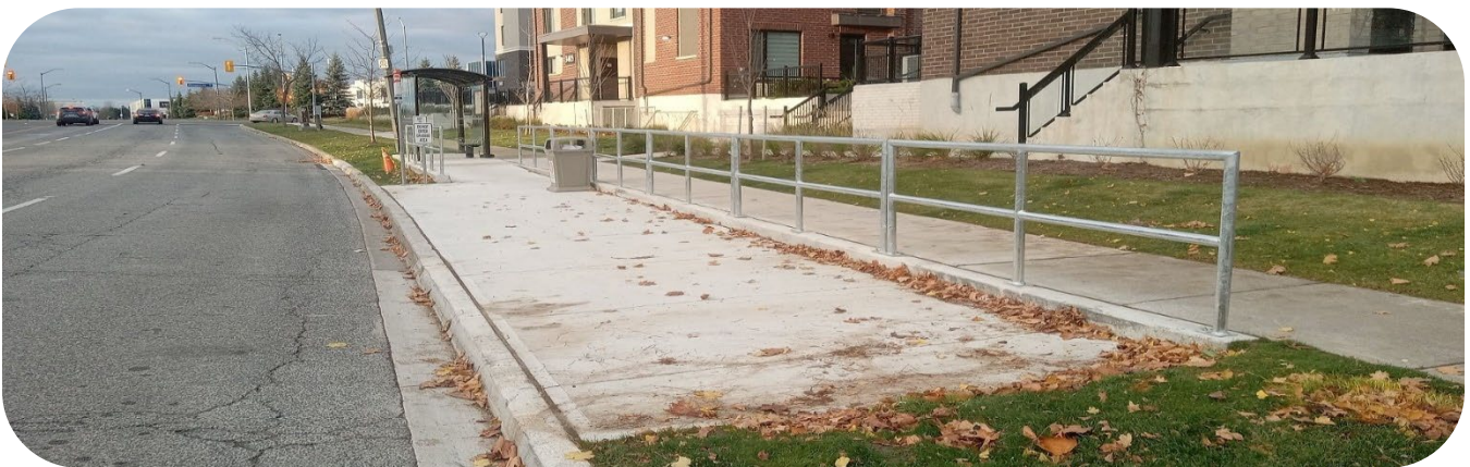
Figure 2: Landing pad with ramp connection at bus stop#0527 The Collegeway at Ridgeway Dr. that meets the slope requirements.
