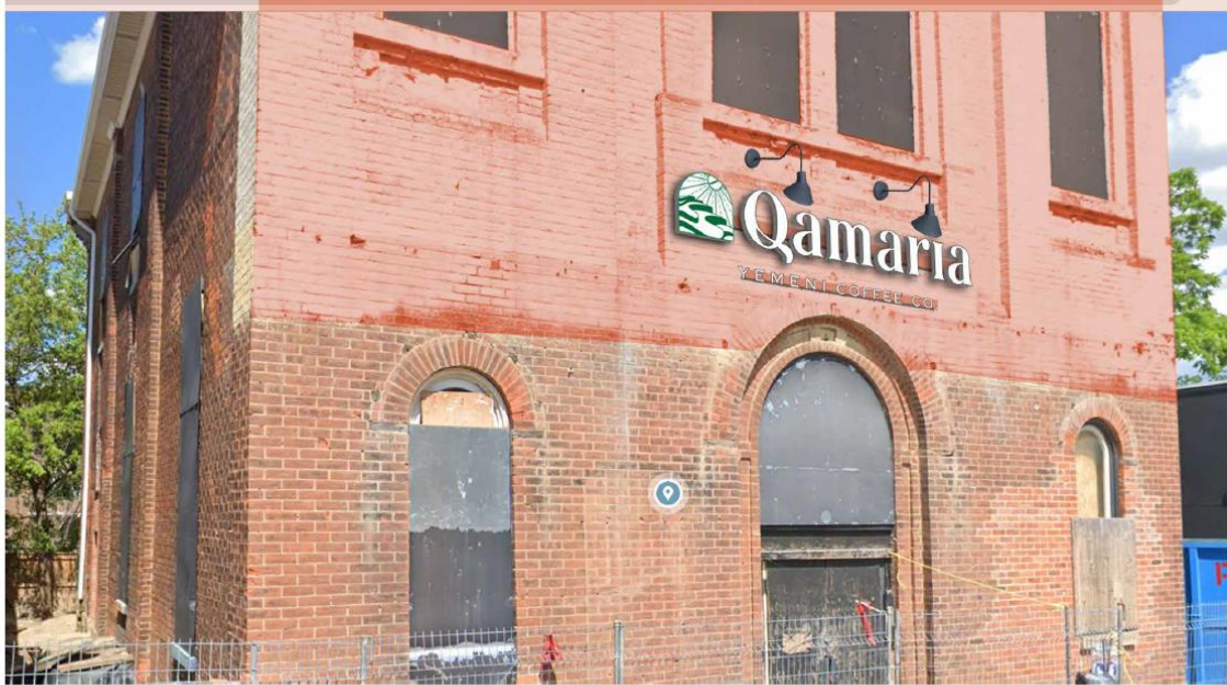
North Side Front Entrance
