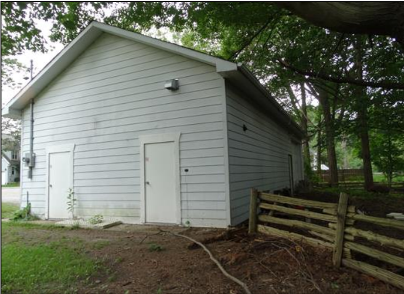
Figure 3: North and west (R) facades of garage, 2017
