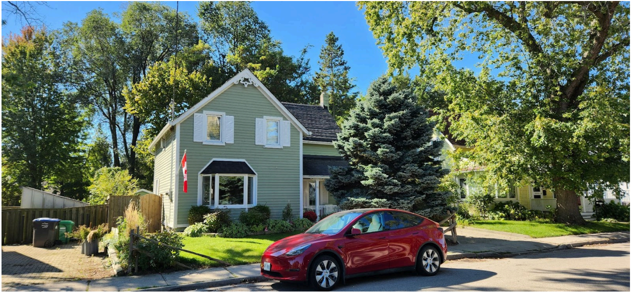
Figure 2: 42 John Street South viewed from the east, showing sage green painted clapboard cladding; white trim, shutter, and flourishes; and grey asphalt shingles. (Photo by owner, October 2024)
