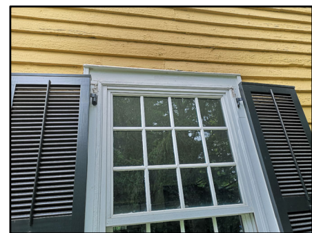
TYPICAL PEELING PAINT, SIDING DETERIORATION
