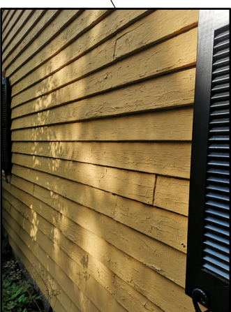
TYPICAL PEELING PAINT, SIDING DETERIORATION
