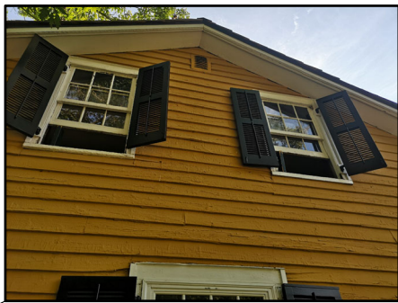
TYPICAL PEELING PAINT, SIDING DETERIORATION
