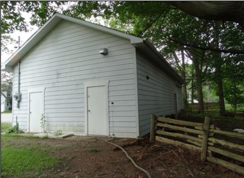
Figure 3: North and west (R) facades of garage, 2017
