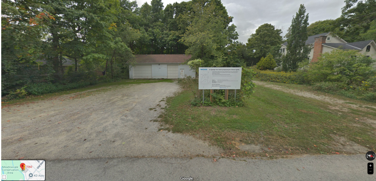
Photo 5: Existing streetscape 7060 Old Mill Lane. 7050 Old Mill Lane is not visible and only a portion of 7070 Old Mill Lane is visible.
