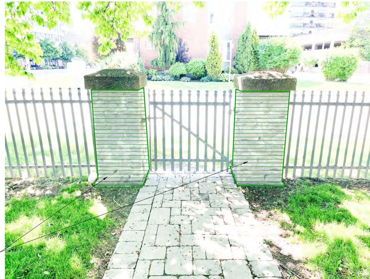
SOUTH STONE PIERS - NORTH ELEVATION
