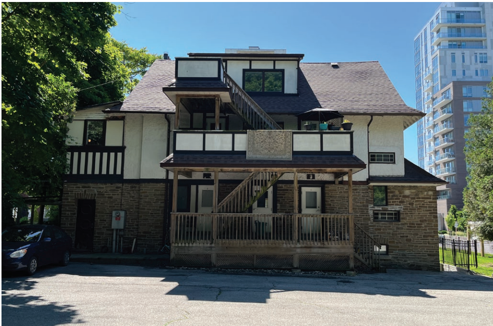
Rear (north) elevation of 84 High Street East (ERA, 2024).
