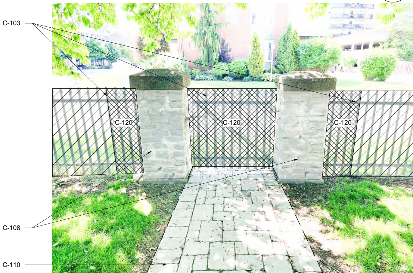
SOUTH STONE PIERS - NORTH ELEVATION
