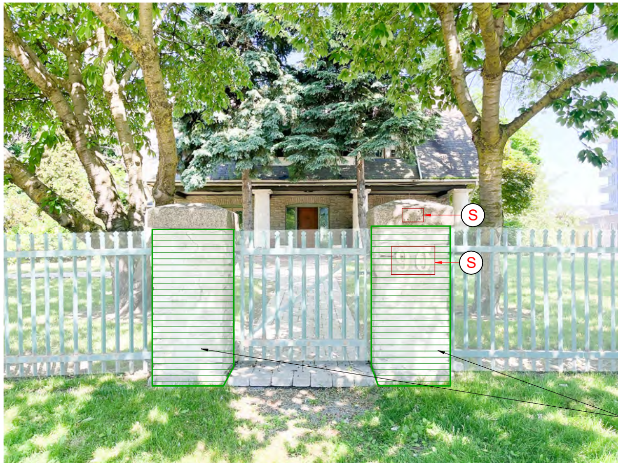
SOUTH STONE PIERS - SOUTH ELEVATION
