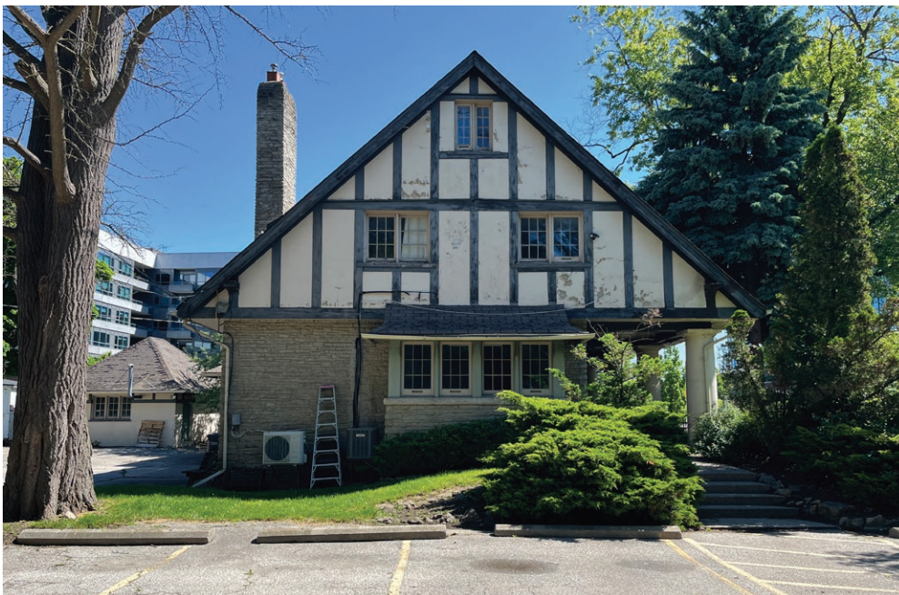
West elevation of 90 High Street East (ERA, 2024).
