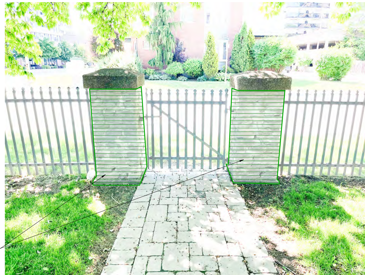
SOUTH STONE PIERS - NORTH ELEVATION
