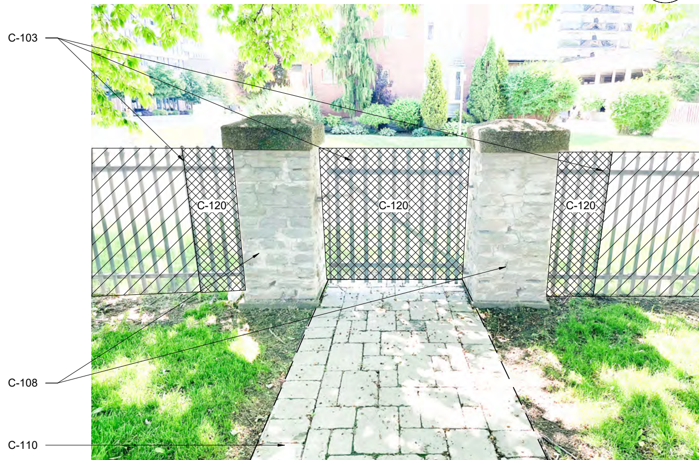
SOUTH STONE PIERS - NORTH ELEVATION
