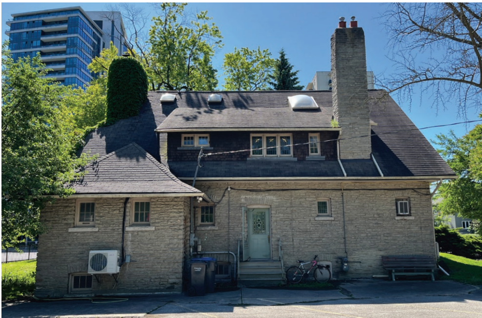
Rear (north) elevation of 90 High Street East (ERA, 2024).
