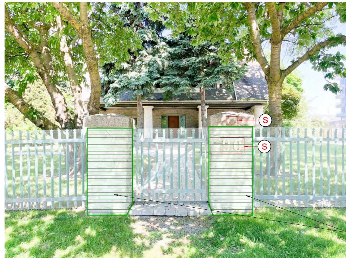
SOUTH STONE PIERS - SOUTH ELEVATION
