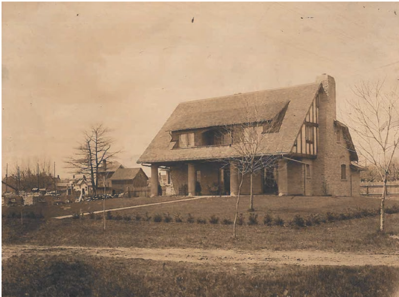
Undated photograph of 90 High Street East, looking northwestward towards the principal (south) elevation (FRAM + Slokker).
