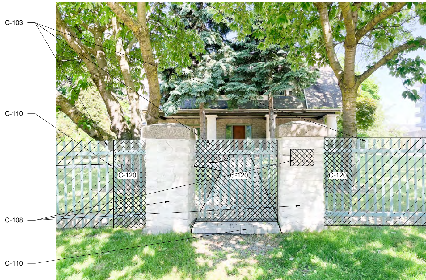
SOUTH STONE PIERS - SOUTH ELEVATION
