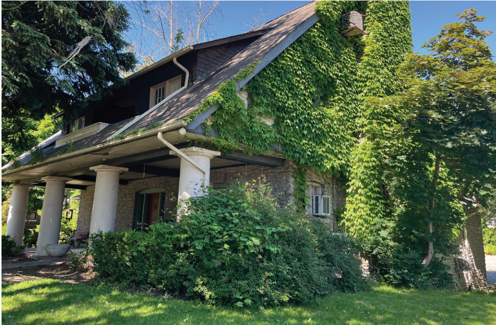
Primary (south) elevation and east elevation of 90 High Street East (ERA, 2024).
