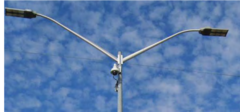
CCTV Camera mounted on Street Light Pole
