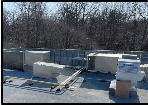
Heat Pump Roof Top Units (4 Facilities)
