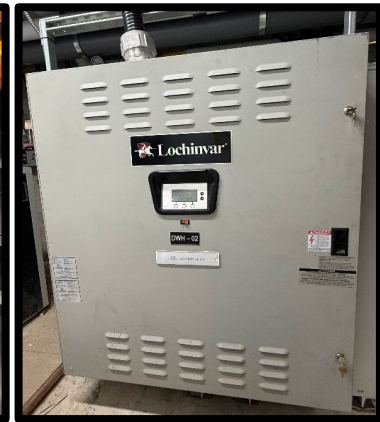
Electric DHW boiler (Hybrid System)
