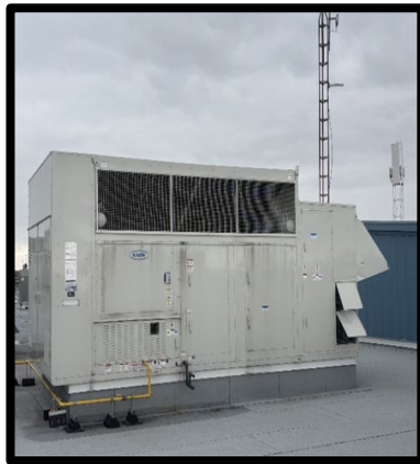
Air Sourced Heat Pump MAU
