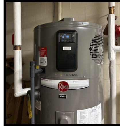
Heat Pump Water Heater (2 Facilities)
