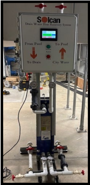
Pool Drain Heat Recovery (2 Systems at 1 Facility)
