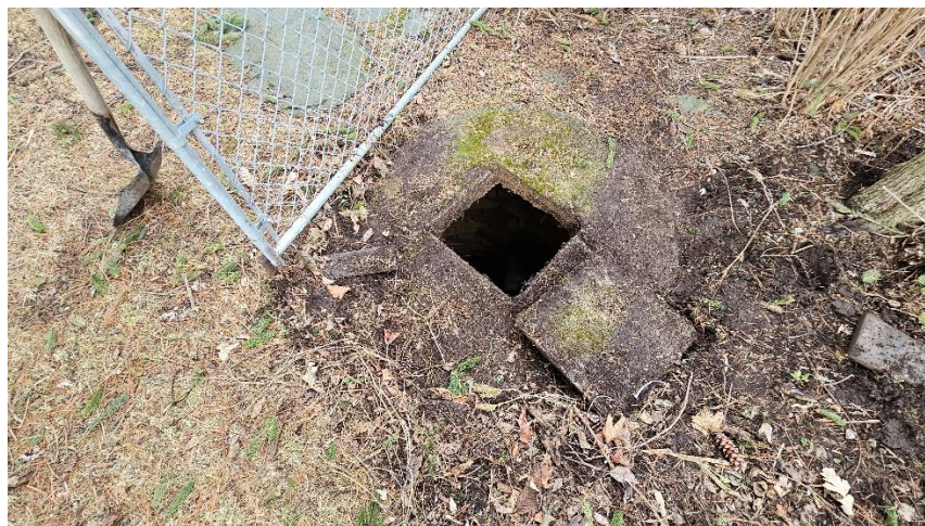
Photograph 6: Cistern Exterior Surface
