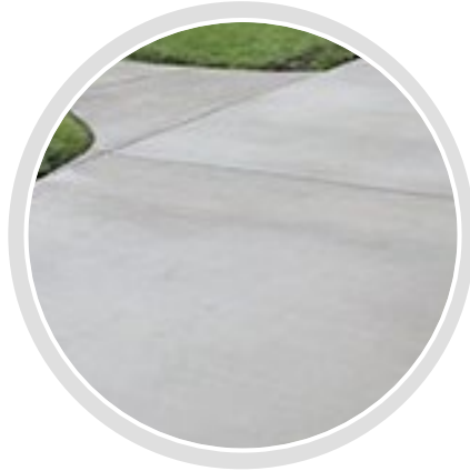
Concrete Paving PLAZA AND WALKWAYS
