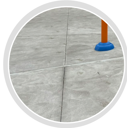
Sandblasted Concrete SPRAY PAD
