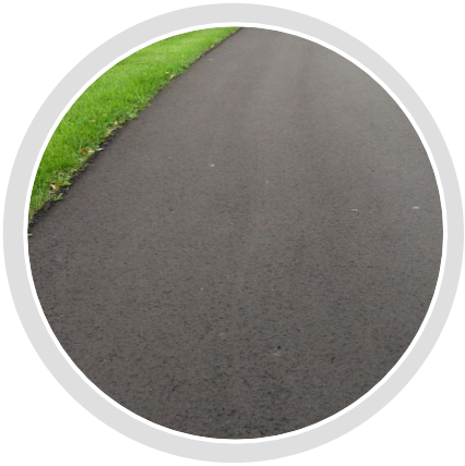
Asphalt Paving WALKWAYS AND TRAILS
