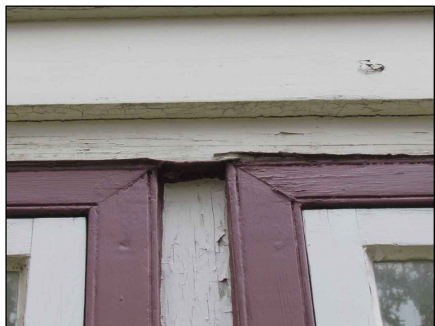
M. DETERIORATED FLASHING ABOVE WINDOWS
