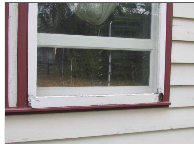
N. DETERIORATED STORM FRAMES
