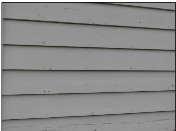
T. SPLIT BOARDS AND RUSTED NAILS
