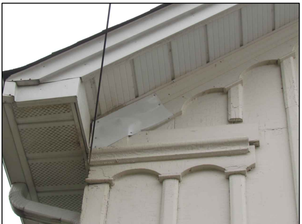
B. DAMAGE TO TOP TRIM
