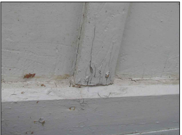
G. DETERIORATION AT BOTTOM OF BOARDS & BATTENS
