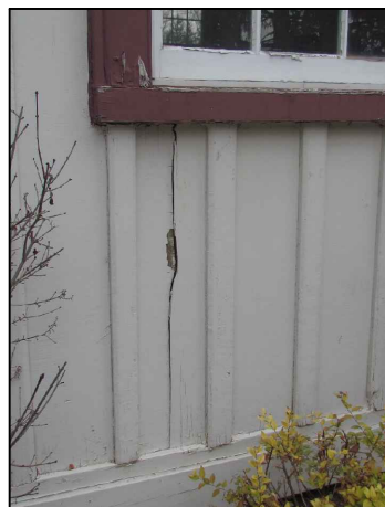
Q. REPLACE CRACKED BOARD
