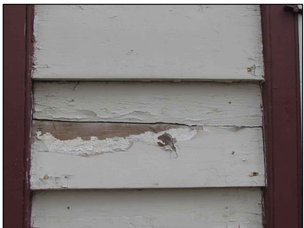
L. BOARDS FOR REPLACEMENT
