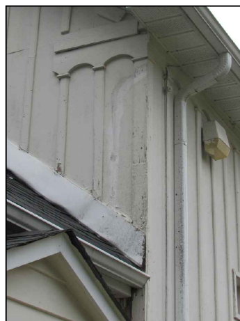
K. CONDITION OF BOARD & BATTEN ABOVE ADDITION'S ROOF, AS WELL AS FLASHING
