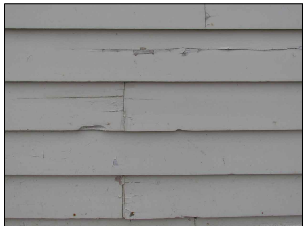
J. CRACKED BOARDS & DETERIORATED BOARDS' ENDS
