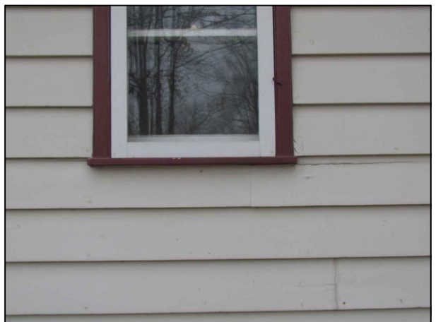
I. WINDOW SILL & CRACKED BOARDS
