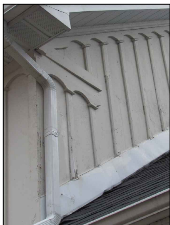
K. CONDITION OF BOARD & BATTEN ABOVE ADDITION'S ROOF, AS WELL AS FLASHING
