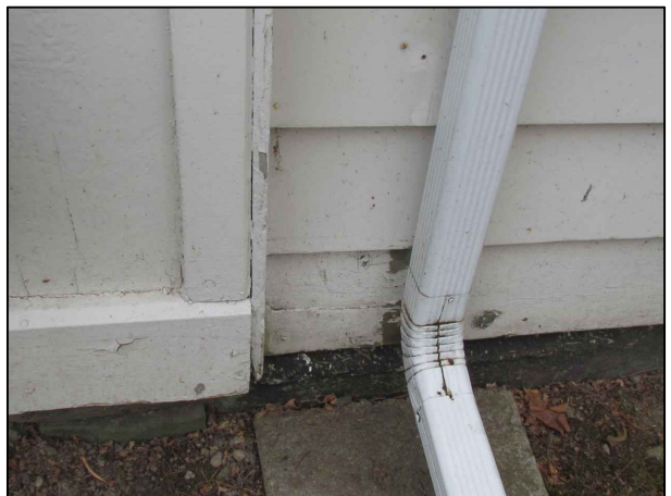
H. DETERIORATION AT BOTTOM BOARD & SKIRTING
