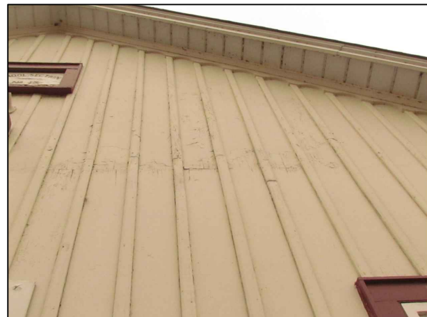
A. DETERIORATION AT BOARDS' ENDS
