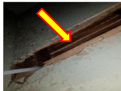
Non-asbestos mortar, Attic space.
