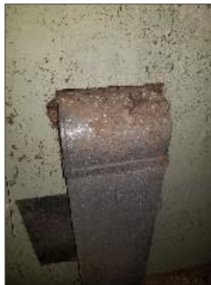
Uninsulated duct, Attic space.
