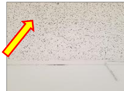
Non-asbestos glued-on ceiling tiles on ceiling, Main Hall, 1 st Floor.
