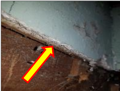
Non-asbestos plaster on wall, Attic space.
