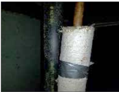
Uninsulated pipe and pipe insulated with fibreglass insulation, Attic space.
