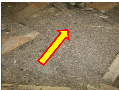
Non-asbestos blown-in attic insulation.
