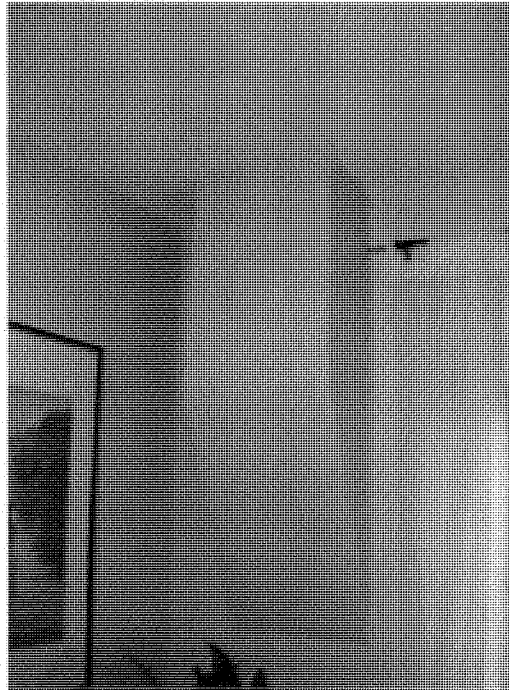
Obsolete and improperly supported chimney
