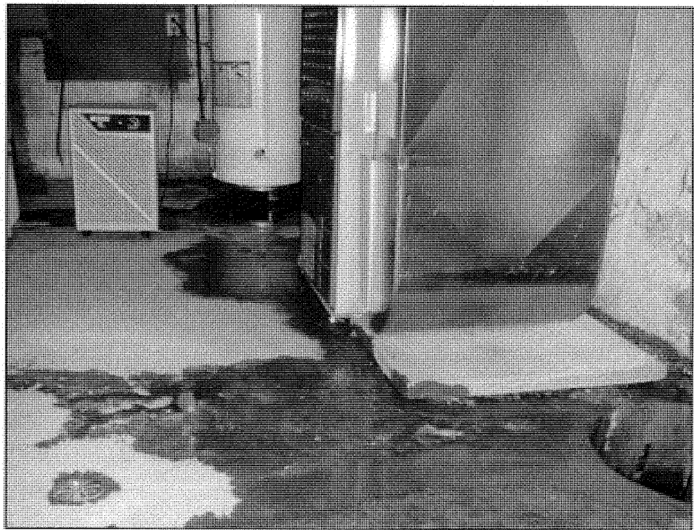
Groundwater seepage in the basement.
