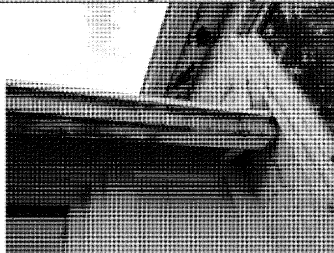
Photo 10: Poor drainage at Eavestrough
