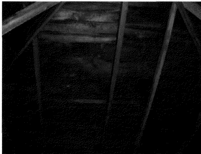
Inadequate and randomly spaced rafters
