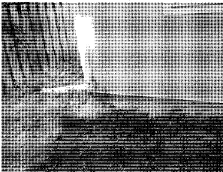
Rear addition with improper foundation and moisture protection
