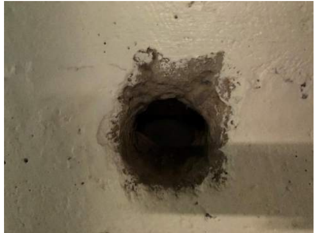
Image 52: View of the hole in the concrete wall revealing concrete construction of the foundation wall.
