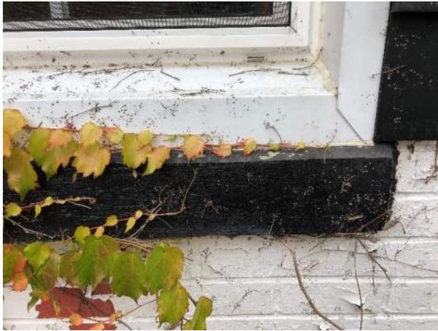
Image 13: Detail of the window surround and sill, note paint wear revealing concrete underneath.
