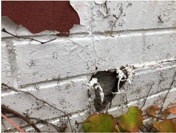
Image 7: Detail of the red-brick veneer peeling away from the concrete foundation.
