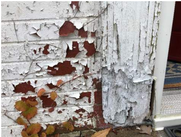
Image 11: Detail of the pilasters, constructed of MDF, around the front door.
