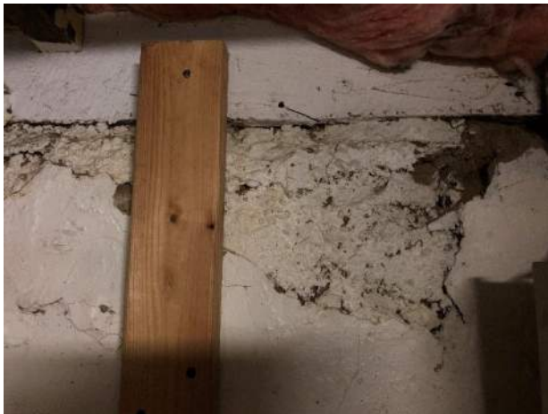
Image 51: View of the concrete foundation, note there was no evidence of stone construction.
