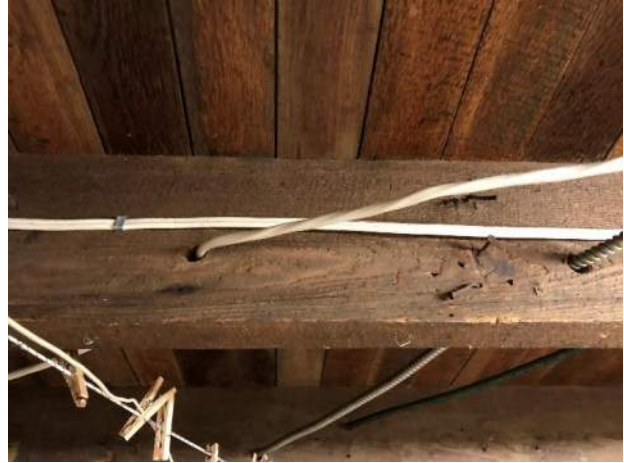
Image 50: View of the machine hewed floor joists.
