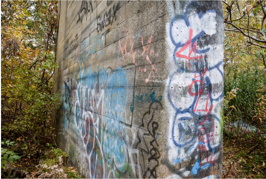
Fig. 72 Detail showing striations in the backstop's poured concrete
