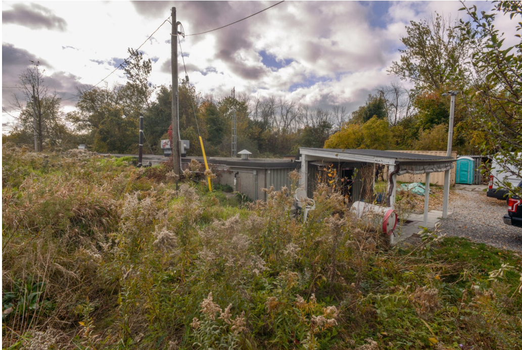
Fig. 48 Corner view of the Indoor Rifle Range, showing the east elevation buried in the ground and the front (north) elevation with a shed-roofed wooden porch added on
