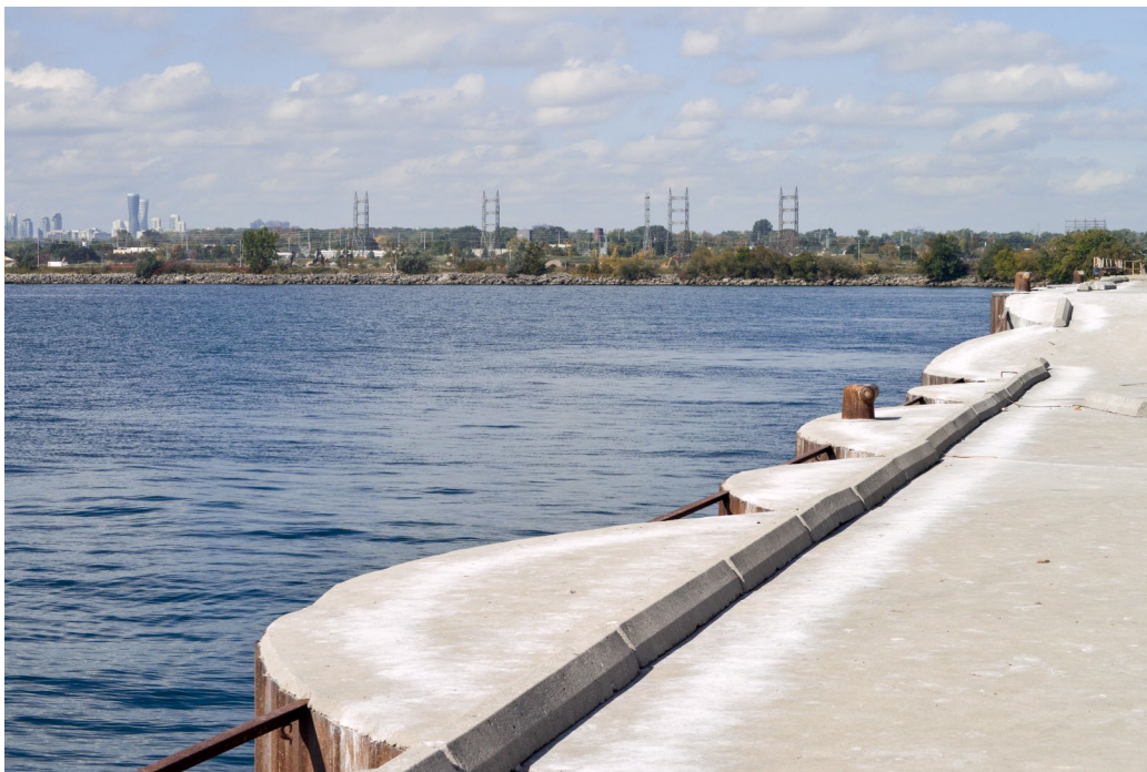
Fig. 39 View on the docking causeway near its south end, looking northwest to the site's transmission towers and beyond to the towers of Uptown Mississauga. Note how the docking causeway's cylindrical-shaped steel cells form a series of arcs along its edge.
