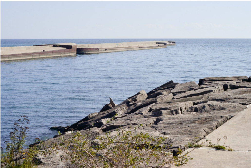
Fig. 35 Another southward view on the docking causeway, showing the intake channel. In this view, on the far left, the eastern breakwater is made of concrete-filled steel barges. In the foreground, the western breakwater for the docking causeway is constructed of boulders.
