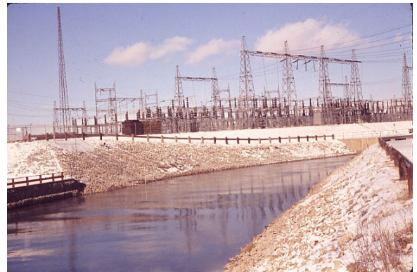
Fig. 17 Ralph Crysler, "Lakeview Generating Station, Discharge," 1972, City of Mississauga Historic Images Gallery, Lakeview Gallery, LG_R141.jpg. The discharge channel is in the foreground, and the switch yard is in the background.
