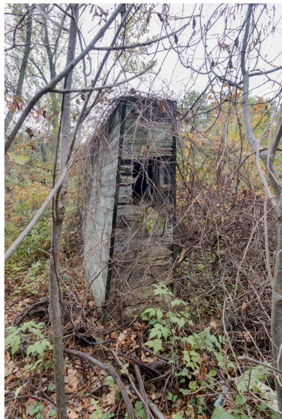
Fig. 59 Northernmost baffle in collection of baffles at Outdoor Firing Range. Note the rectangular hole revealing sand inside the baffle's cavity.
