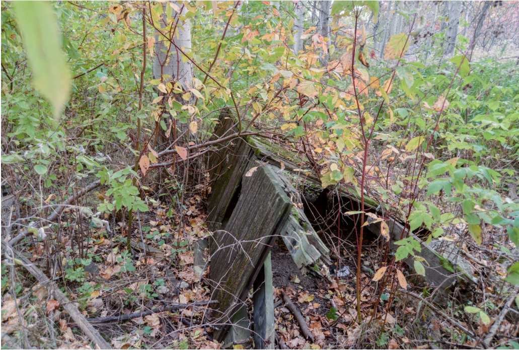
Fig. 66 A collapsed baffle found in the bush
