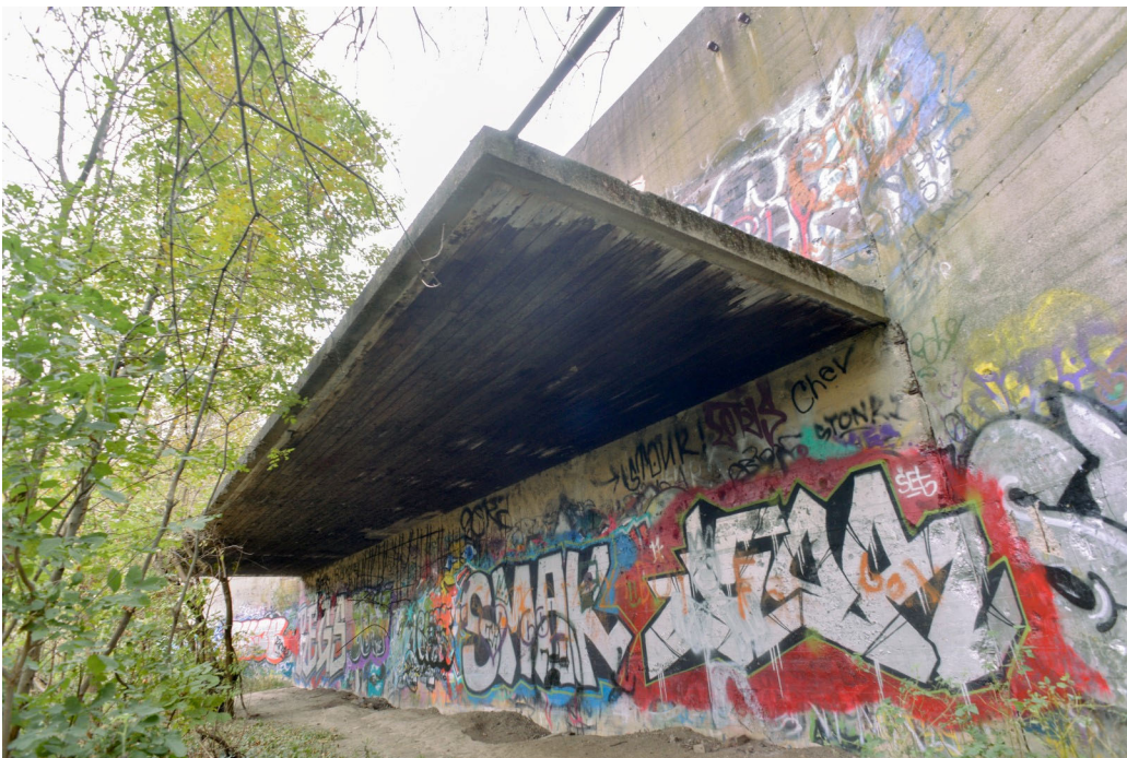
Fig. 69 Canopy on north face of backstop. The canopy is formed of concrete and has a wooden underside. Graffiti has been sprayed on the lower portion of the backstop's concrete wall and above the canopy.
