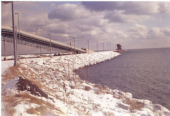
Fig. 16 Ralph Crysler, "Lakeview Generating Station Pier," 1972, City of Mississauga Historic Images Gallery, Lakeview Gallery, LG_R169.jpg. Note the truss structure of the elevated coal conveyor.
