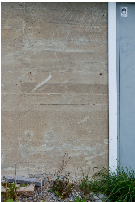
Fig. 51 Detail of the west elevation's concrete wall, clearly showing the striations of poured concrete
