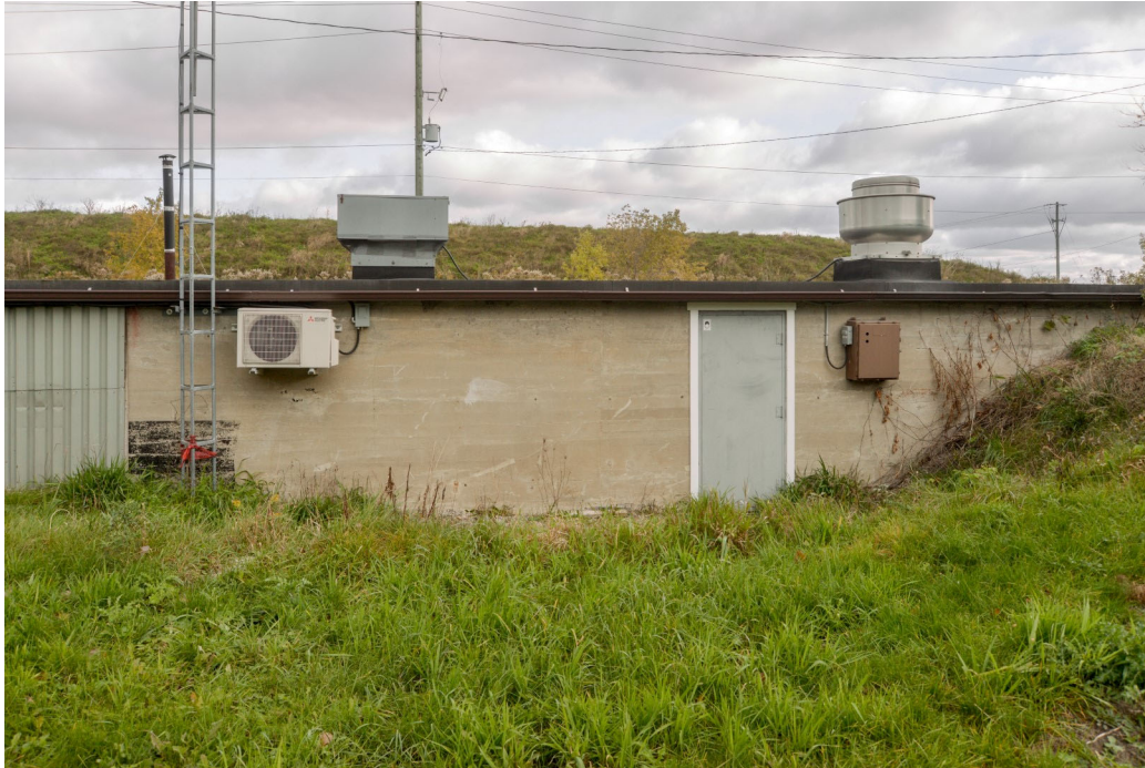
Fig. 50 Detail of the west elevation, showing corrugated metal cladding on the left and the range's exposed concrete construction on the right
