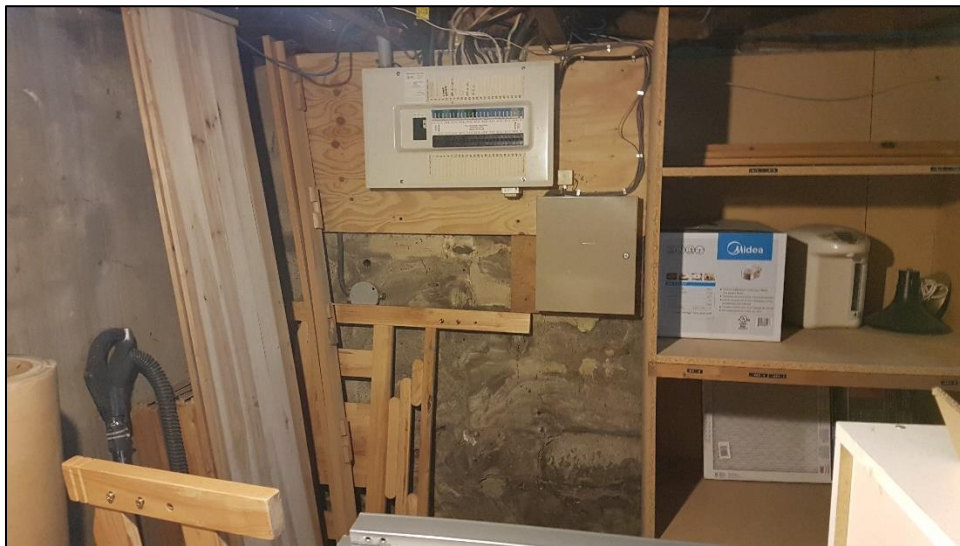
Figure 73: Basement photo showing the concrete block foundation with parging
