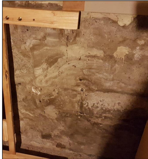
Figure 85: Concrete block foundation with parging
