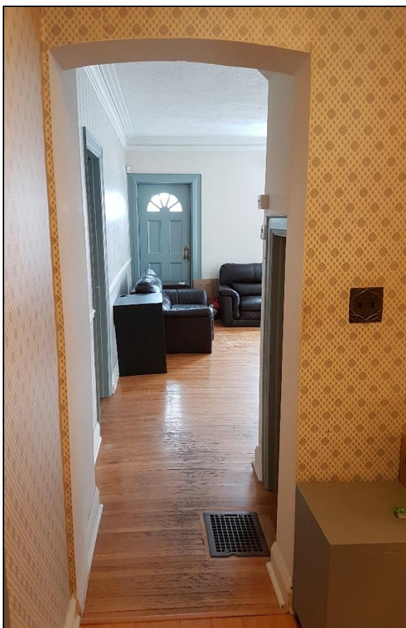
Figure 54: Connection between the original building and rear addition
