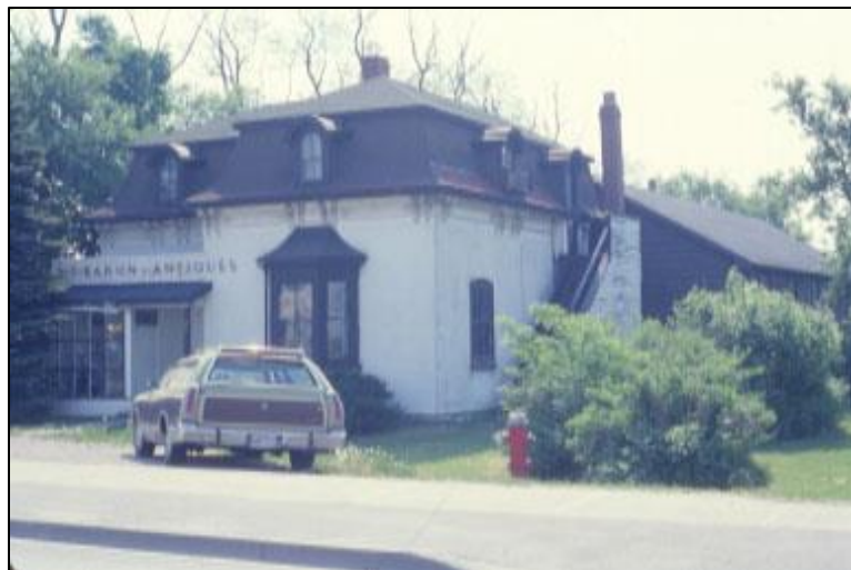
Figure 77: 264 Dundas Street East (Mississauga Library LG_A690)
