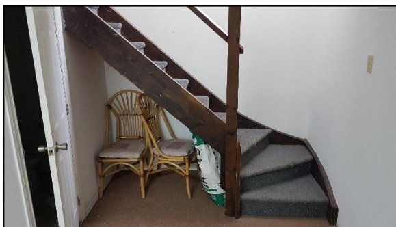
Figure 69: Staircase to the basement
