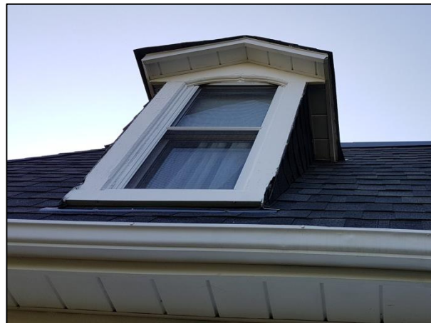
Figure 35: Second storey dormer
