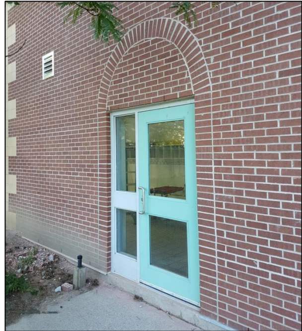
Figure 28: Brick arch above the north elevation doors
