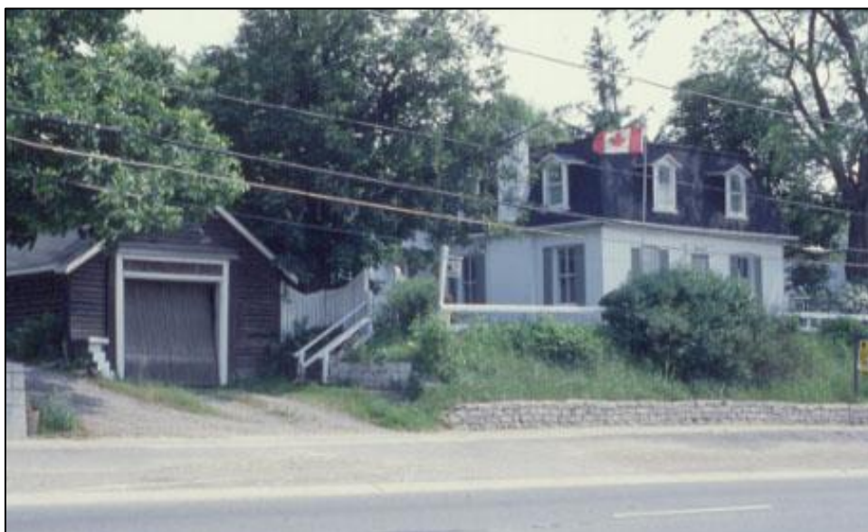
Figure 11: Taylor-Froebel House c.1978 (Mississauga Library B529)
