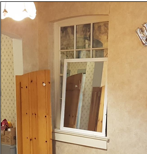
Figure 86: Photo of an original rear window, now present within the residence
