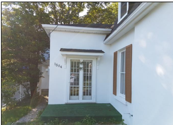
Figure 37: East elevation entrance
