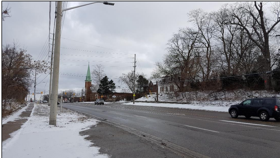
Figure 74: Eastward view along Dundas Street West
