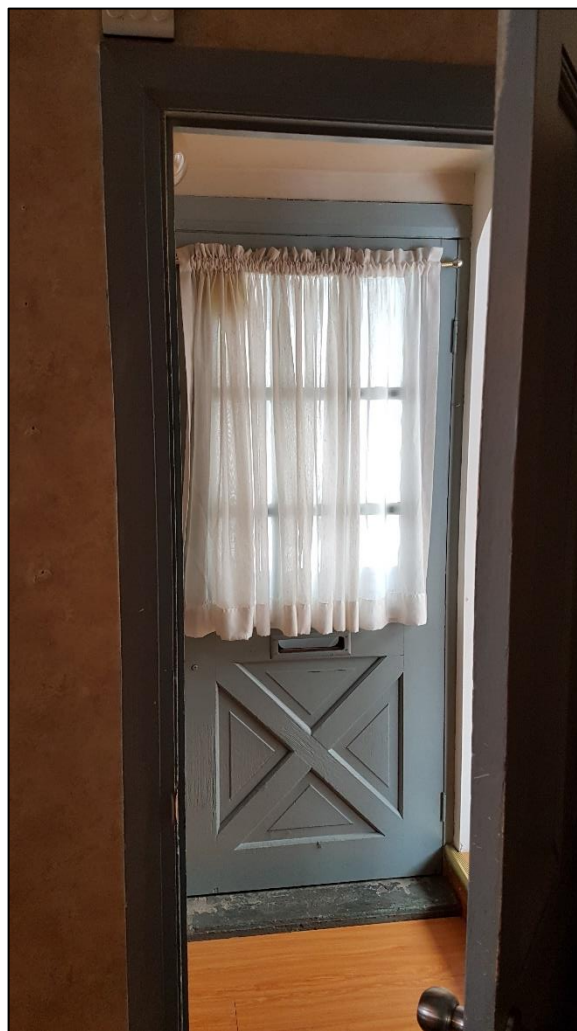
Figure 61: Secondary entrance door on the east elevation
