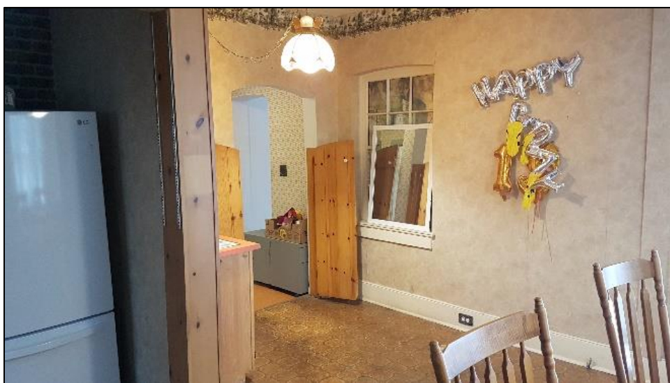
Figure 59: Kitchen, showing one of the original building's original windows
