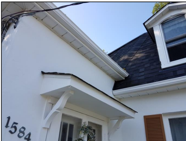
Figure 39: Wooden awning above the side entrance.
