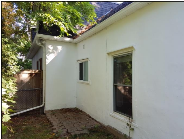
Figure 43: West elevation of rear addition
