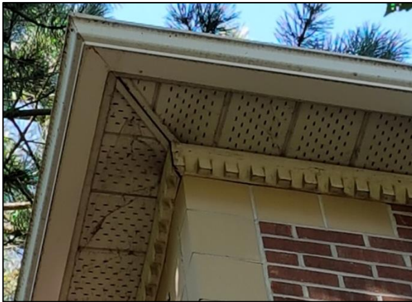
Figure 29: Dentil cornice
