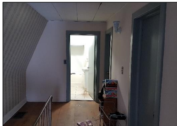
Figure 68: Second floor hallway
