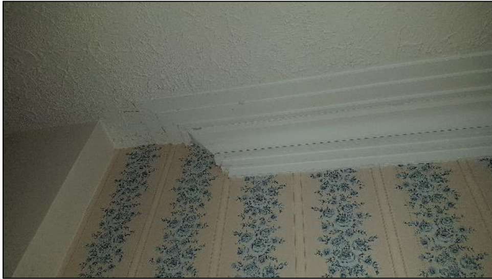
Figure 50: Crown moulding within the front room
