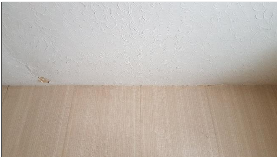
Figure 53: Stucco ceiling in the first floor bedroom
