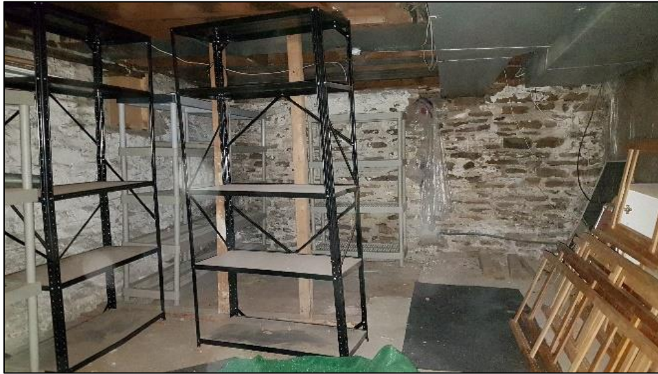
Figure 72: Unfinished basement with stone foundation walls
