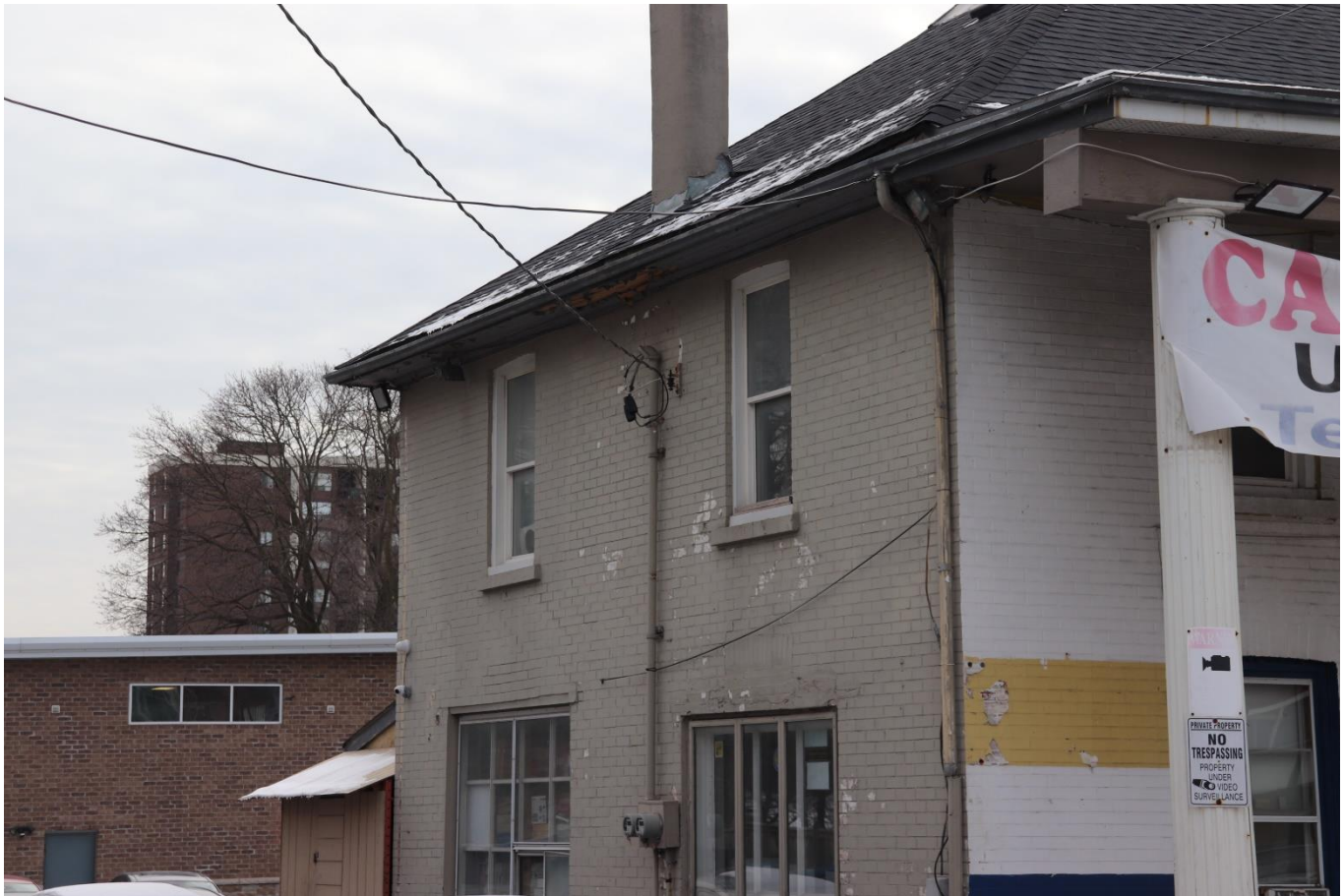
Photograph 12: View of the east elevation illustrating, the two aluminum one-over-one sash window with painted grey concrete sills, looking south (AECOM 2021)
