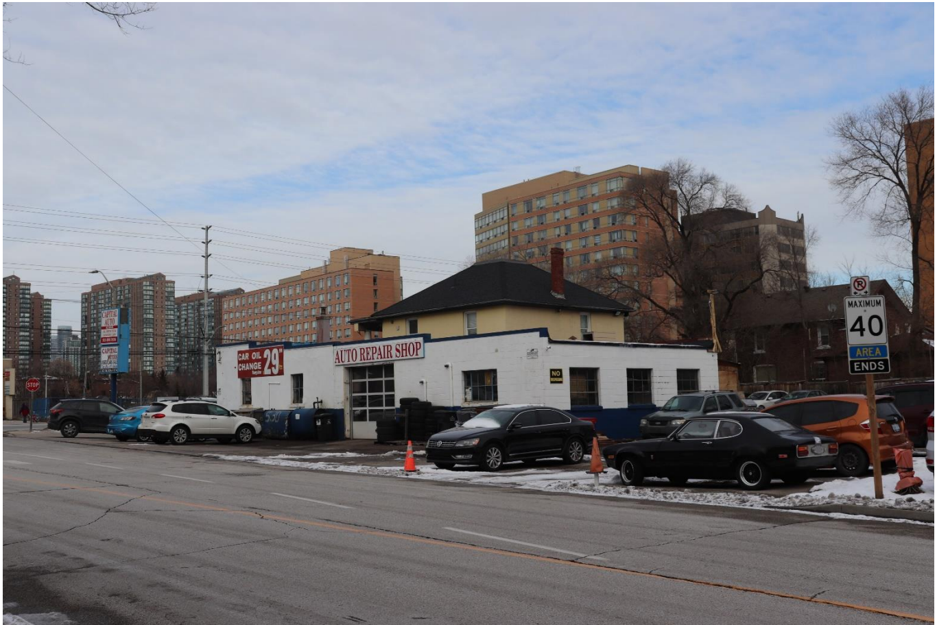
Photograph 8: South elevation (AECOM 2021)
