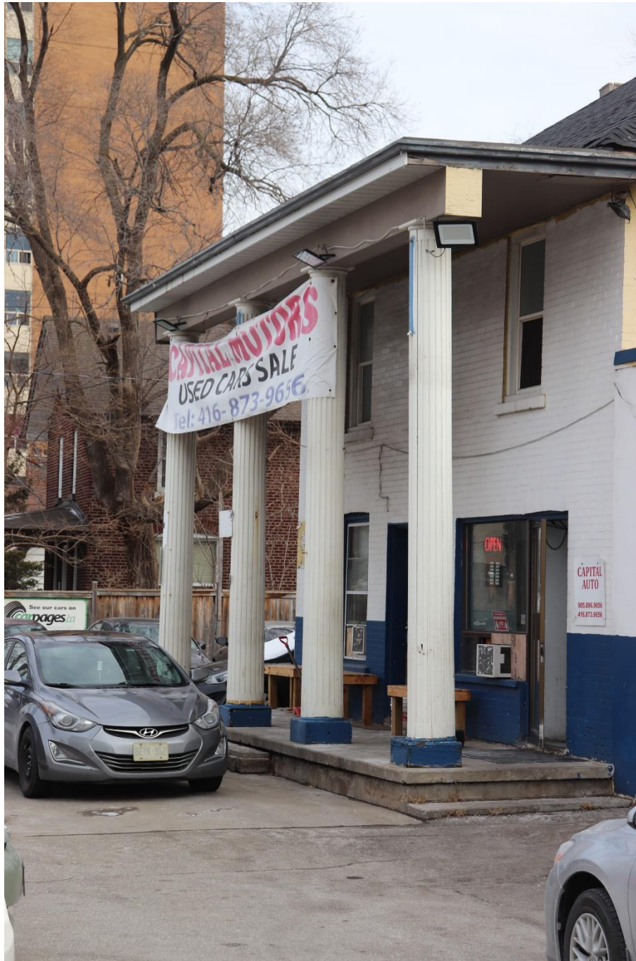
Photograph 2: View of the north elevation, illustrating the double height Doric columns and the concrete porch that spans the length of the elevation, looking east (AECOM 2021)
