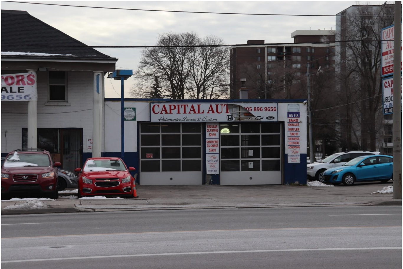
Photograph 4: View of the north elevation, illustrating the attached two-bay automatable service garage, looking south (AECOM 2021)
