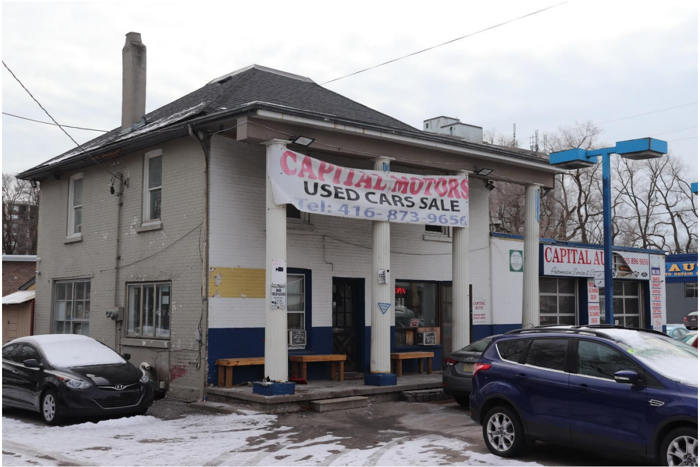
Photograph 10: East elevation (AECOM 2021)
