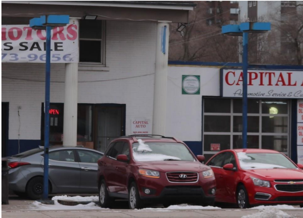
Photograph 5: View of the north elevation, illustrating the concrete slab placed over the dispenser sump and two utilitarian light posts on either side of the concrete slab, looking south (AECOM 2021)
