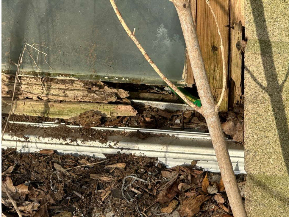
WINDOW DETERIORATION
