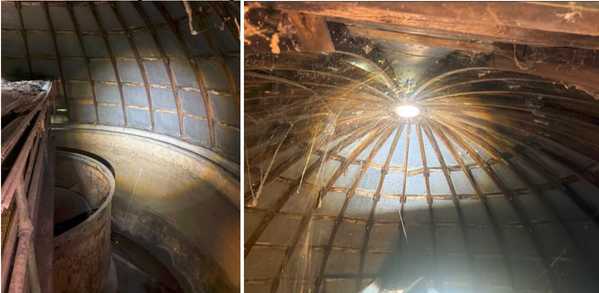
Inside of the existing domical structure planned to be removed.
