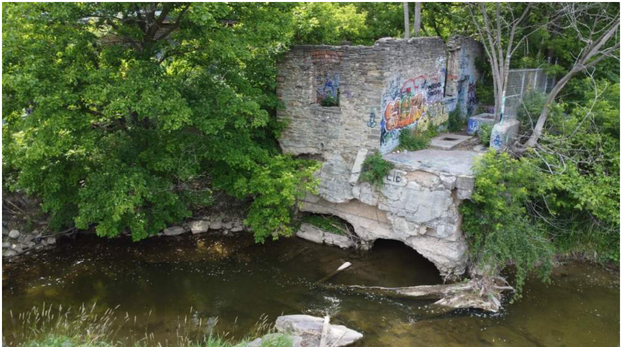
Existing condition of the ruins at the concrete foundation and water discharge and the balcony, on the southeast corner of the building
