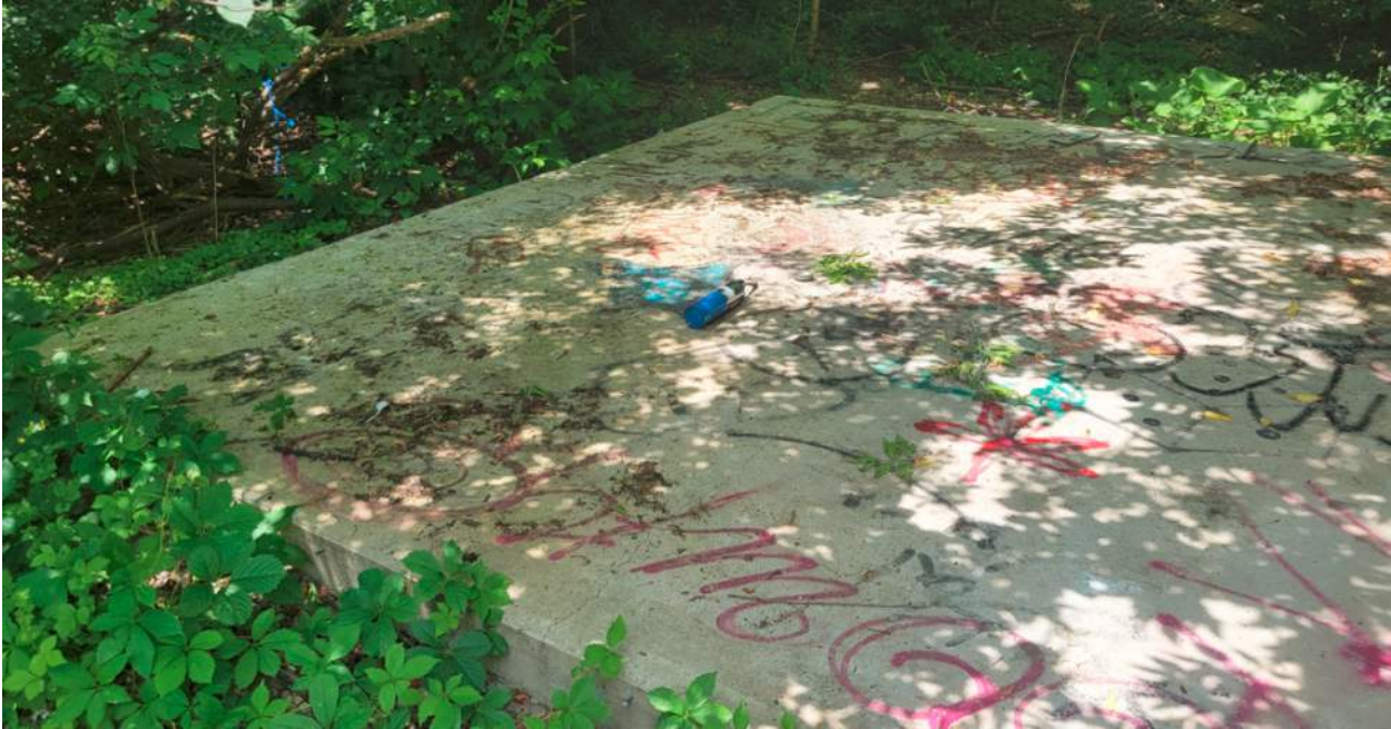
Concrete floor remaining from the Garage
