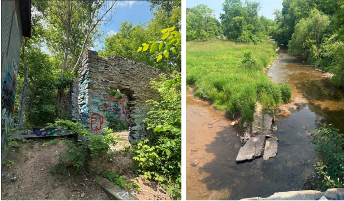
View of the masonry walls (left) and Credit River looking south from the mill (right)
