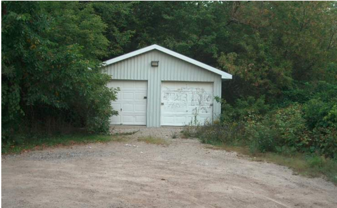
Image of garage prior to demolition of the exterior envelope (image source: 1996 structural report)
