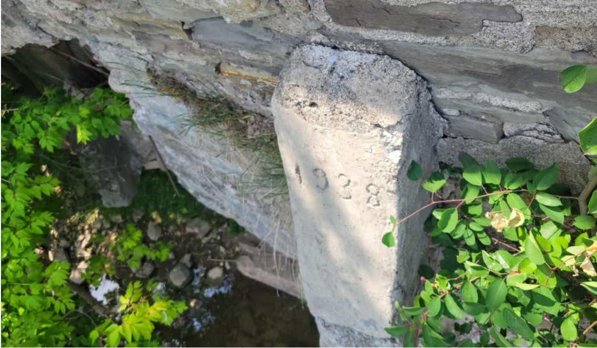
Concrete buttress dated 1938
