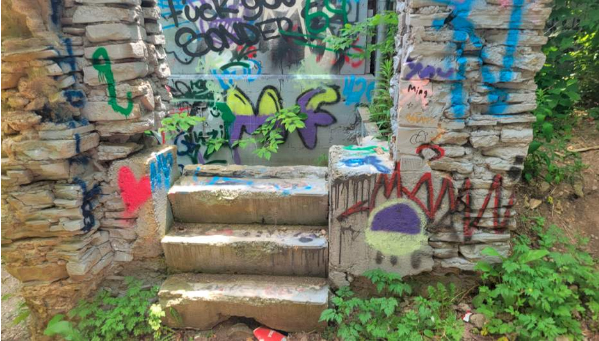
View of the concrete steps
