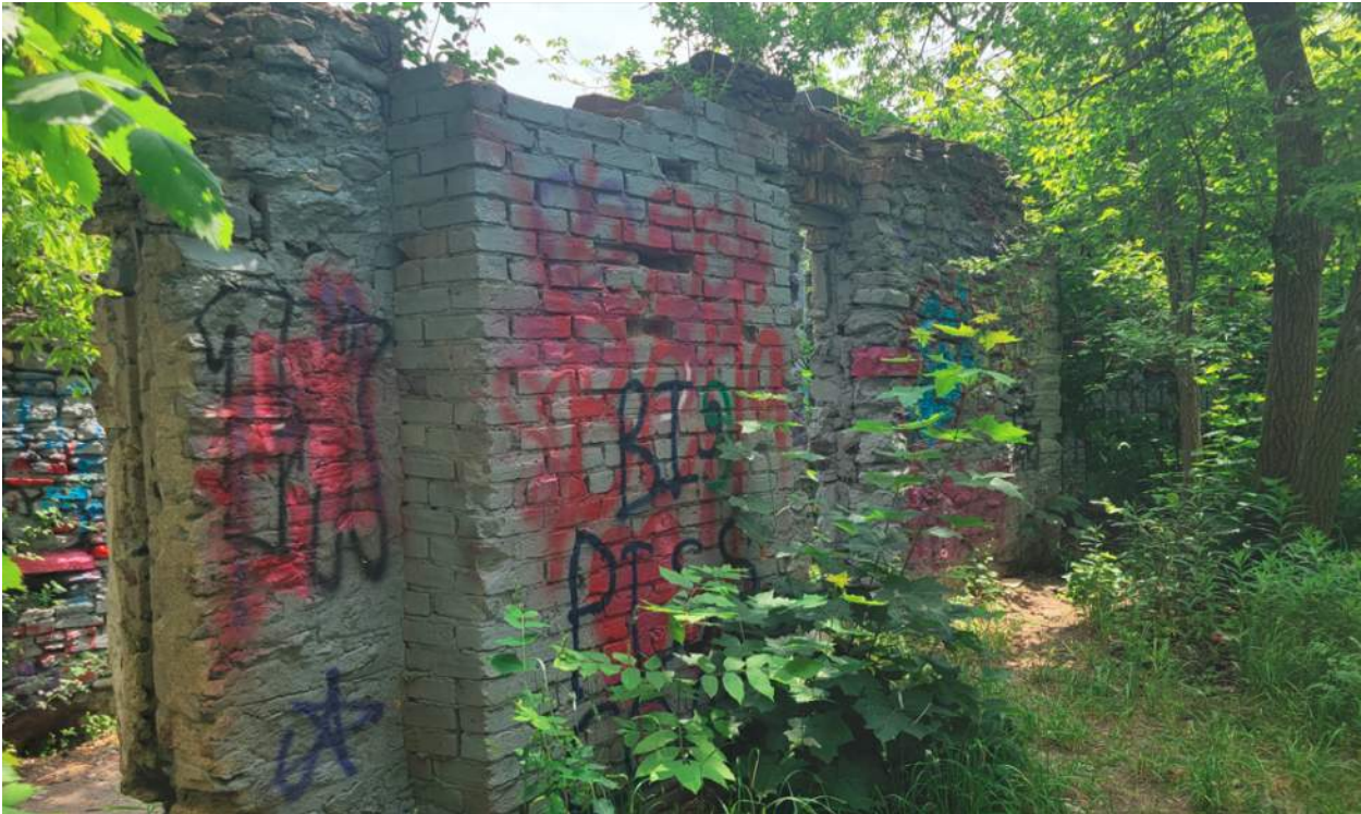
Section of the rubble wall with brick build-out
