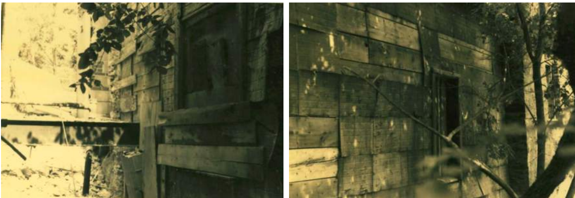
Hyde Mill Ruins (1985) with images of the walls clad with wood (image source: City of Mississauga)
