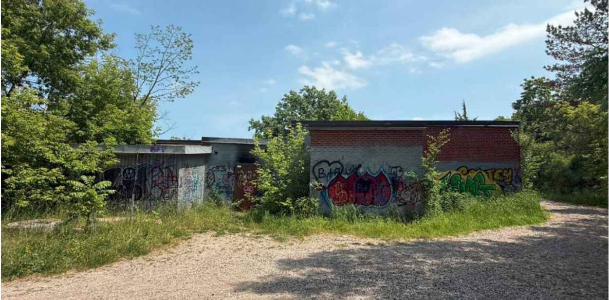
North Elevation of the Pump House Building, with the 1985 washroom addition on the left, clad with concrete veneer blocks
