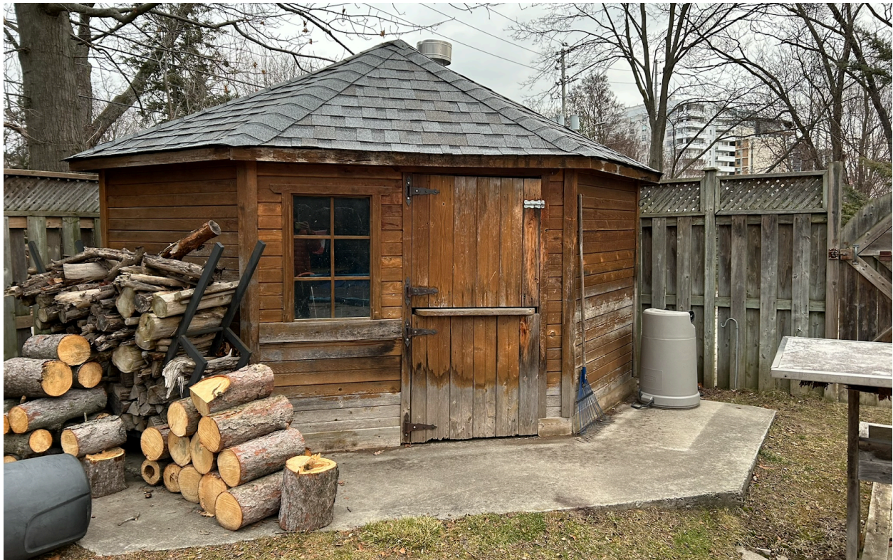
Out building - Pool Equipment
