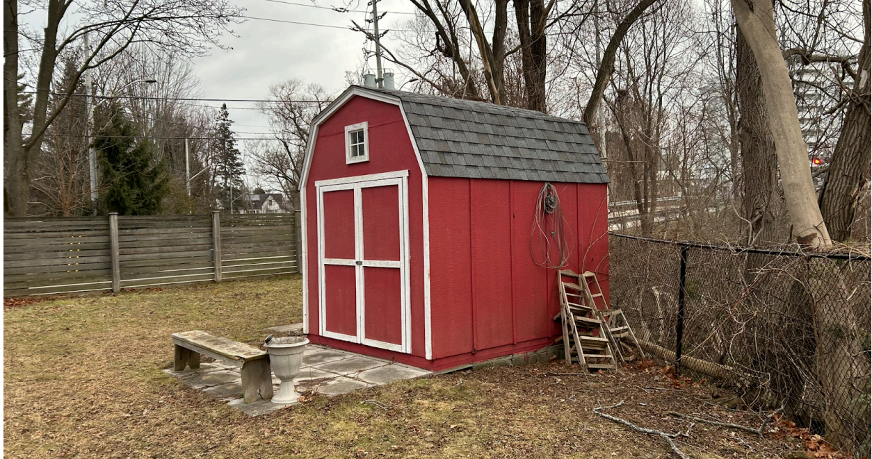
Out building - Shed
