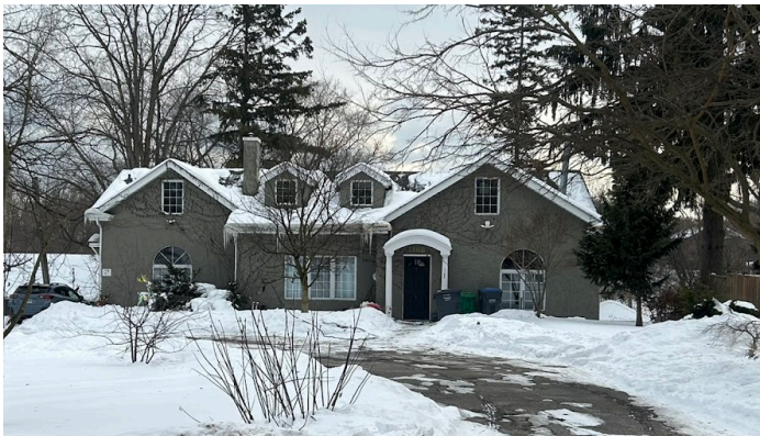
1168 Stavebank Road: stucco duplex.
