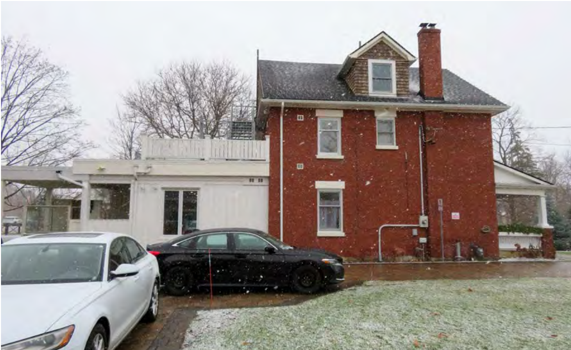
SIDE ELVATION – REAR ADDITION TO BE DEMOLISHED – existing side driveway and parking area
