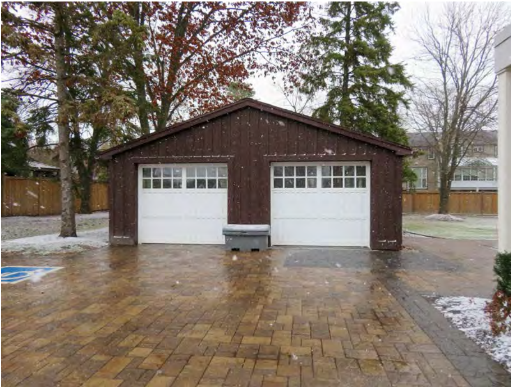
GARAGE – TO BE DEMOLISHED – a modern structure that has no cultural heritage value - concrete pad foundation – board & batten siding, aluminum doors - date of construction estimated to be c.1970s or 1980s
