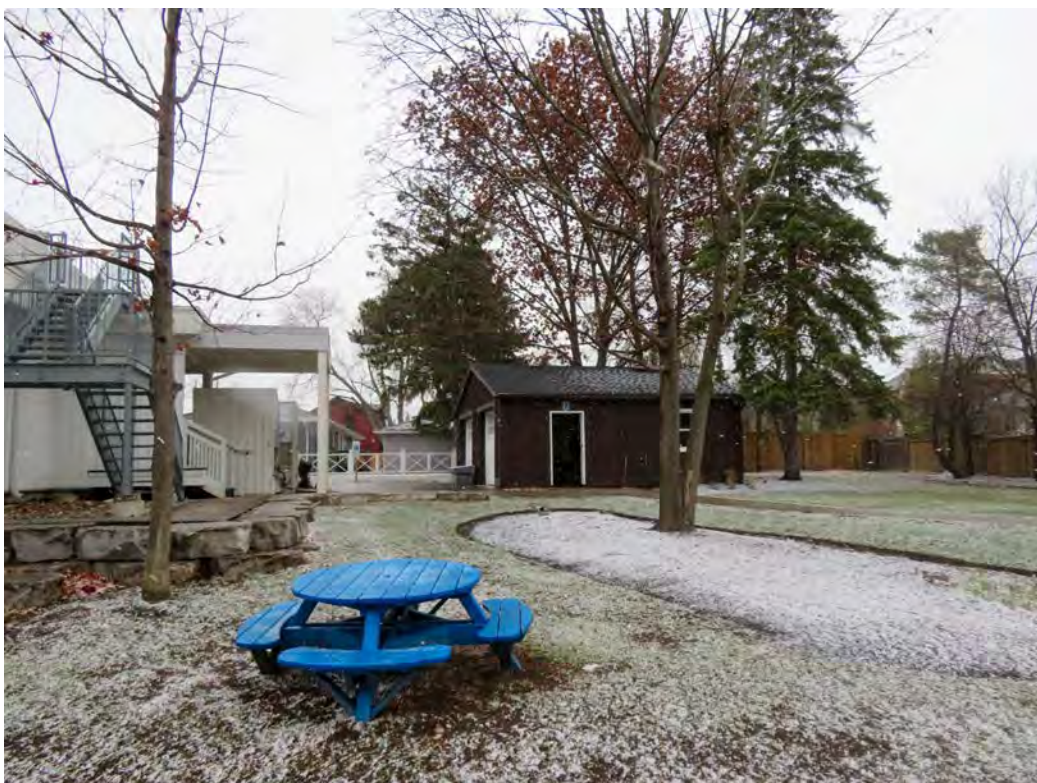
REAR YARD – new rear addition will extend into this space
