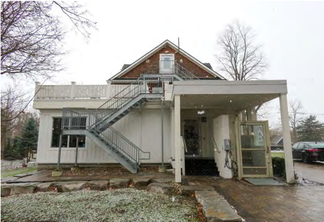
REAR ELEVATION – REAR ADDITION WITH METAL FIRE EXIT AND WHEELCHAIR LIFT TO BE DEMOLISHED
