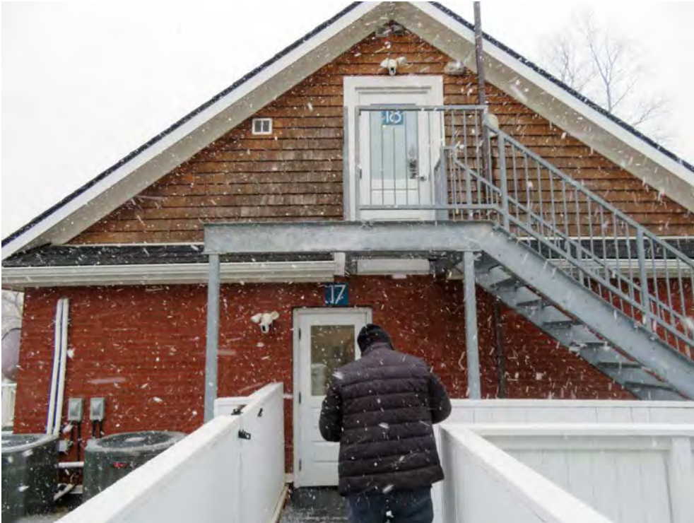
REAR ELEVATION, 2 nd & 3 rd floor level – the exterior brick wall of the house will be retained as a feature wall inside the new addition with new through connections that utilize existing openings – existing a/c units will be relocated
