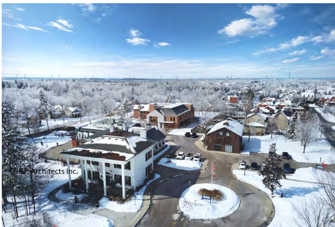
RENDERING – AERIAL VIEW – this view shows the addition within the context of the school campus as a whole and the surrounding residential neighbourhood
