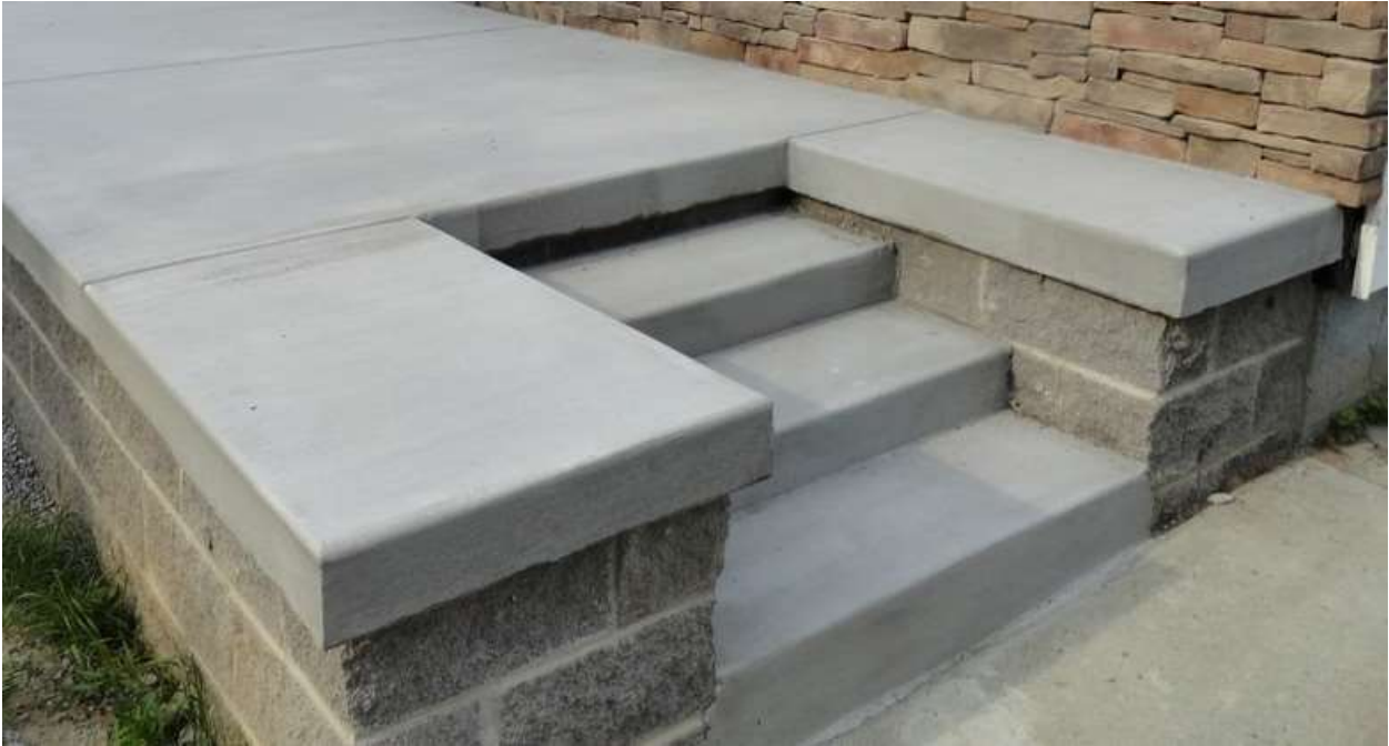
CONCRETE PORCH FLOOR
