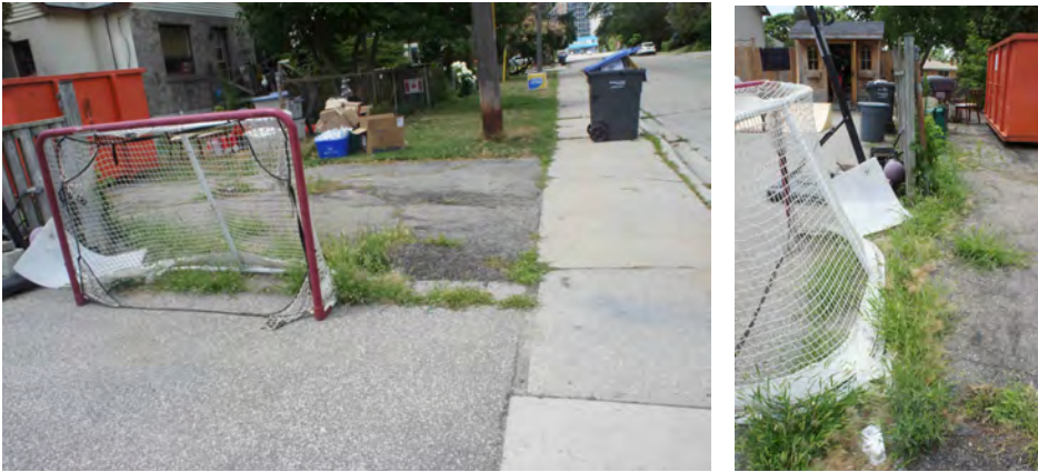
EXISTING DRIVEWAY: opportunity to enhance the District by introducing new landscaping along the edge of the existing driveway
