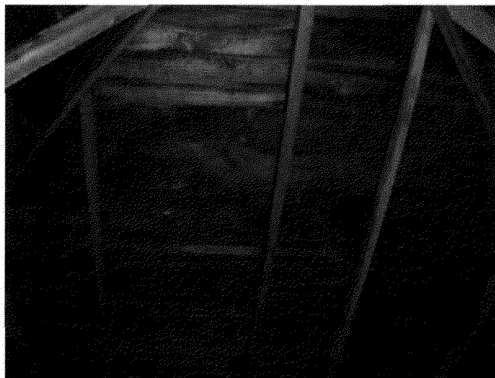
Inadequate and randomly spaced rafters
