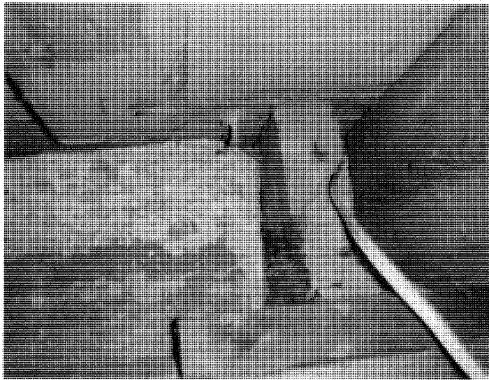
Concrete infill and rotted joist
