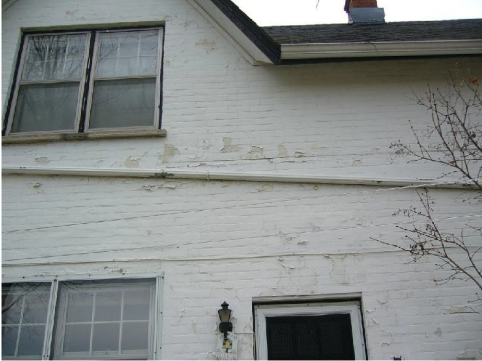
Image 30: Upper and lower windows are enlarged replacements of smaller original windows and openings. Window sills comprise stone units with lintels of steel. The line of a former verandah is discernible above the diagonal drainpipe.
