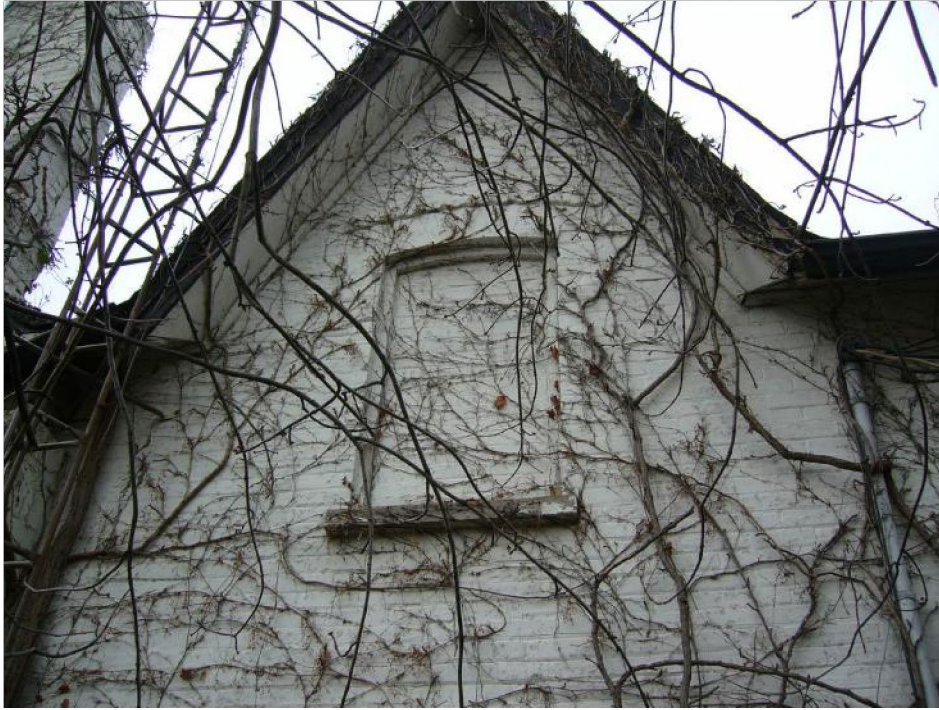
Image 22: Blocked up or “Blind” window second storey
