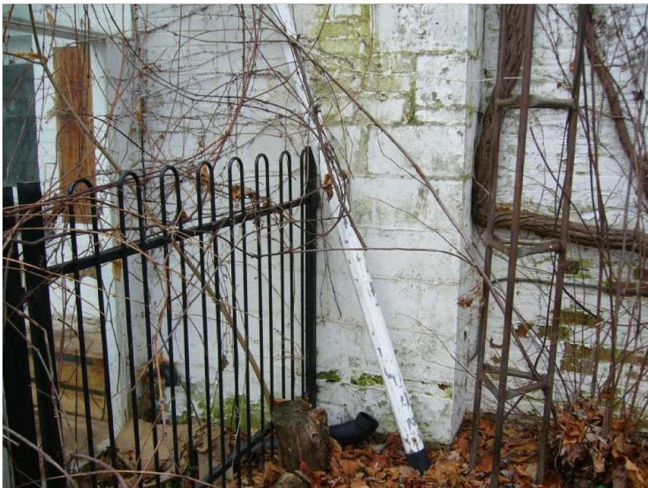
Image 21: Example of exterior degradation resulting from poor maintenance, note disconnected downspout and vegetation growth
