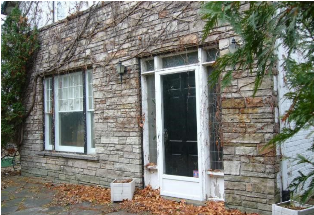
Image 13: Modern tri-partie window and doorway with sidelights and transom on lower level with applied multi-colour stone façade
