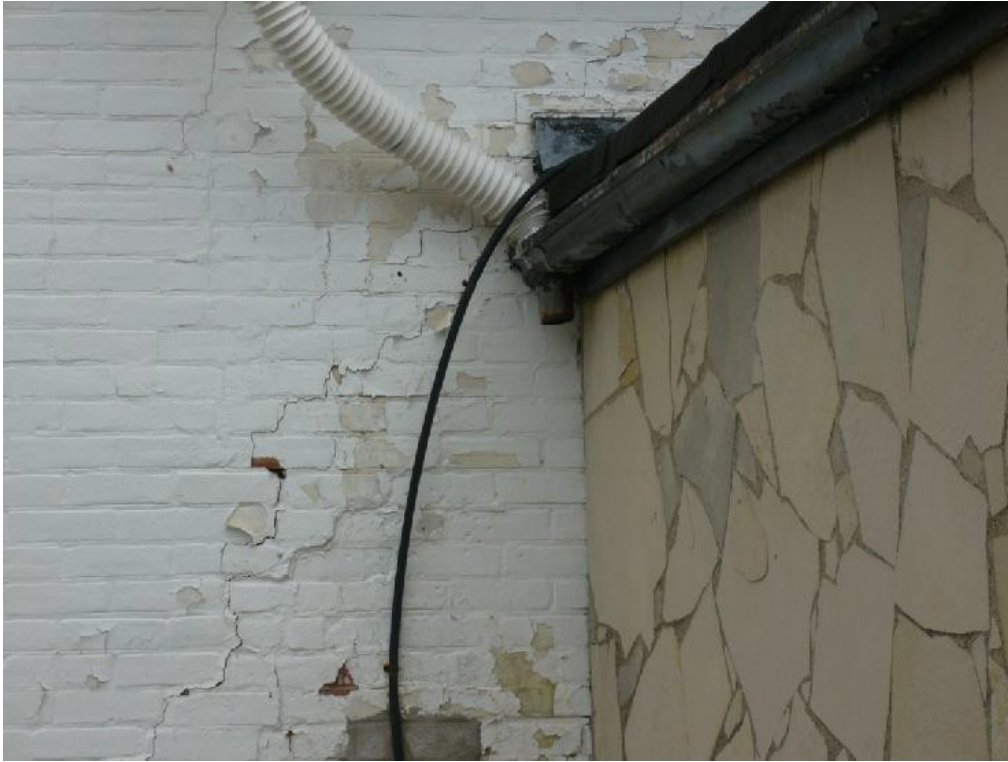
Image 27: Water damage has resulted in cracking of brickwork and mortar joints
