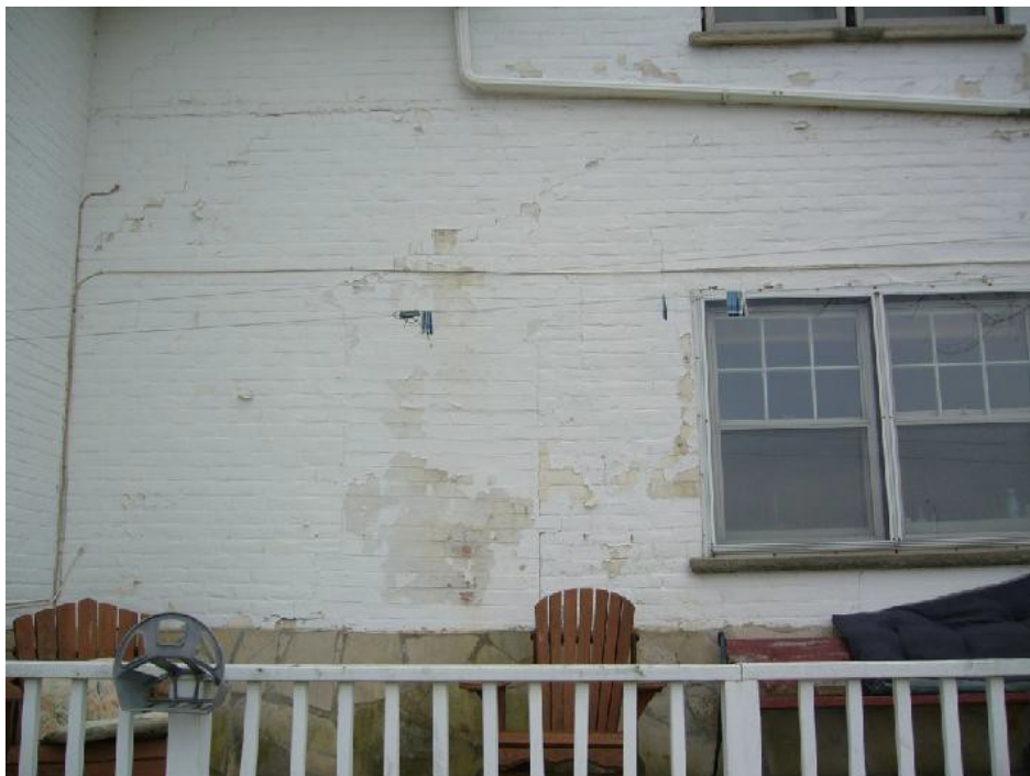
Image 32: An original window opening has been blocked in to the left of the windows. Cracks in the brick work are discernible in the upper corner. Paving has been used to reclad the lower brick courses
