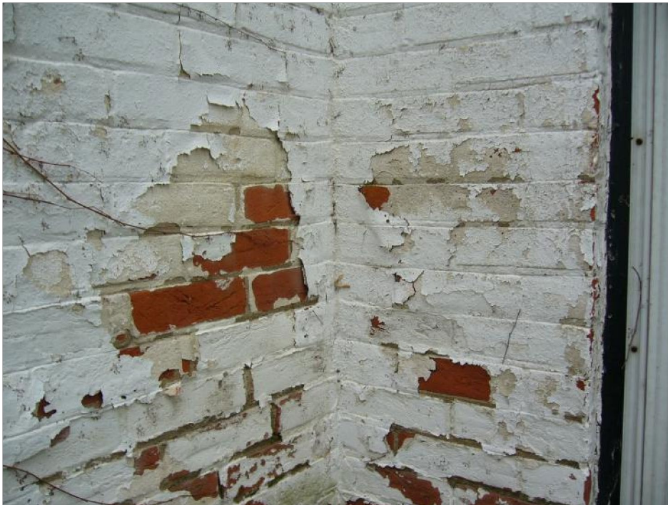
Image 17: Deteriorating paint and cementitious render over original red brick. Interior corner shows aligned brick courses indicating same date of construction.
