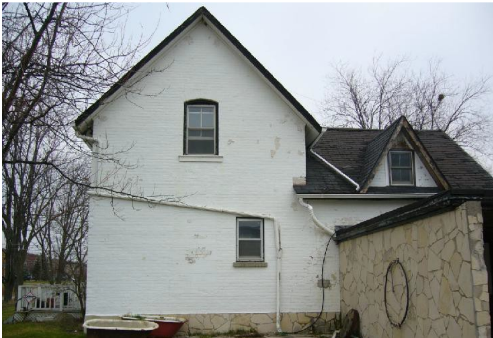
Image 25: West façade showing gable end of 19 th century building and later stone clad carport wall. The lower floor window under the upper floor window has been blocked up.
