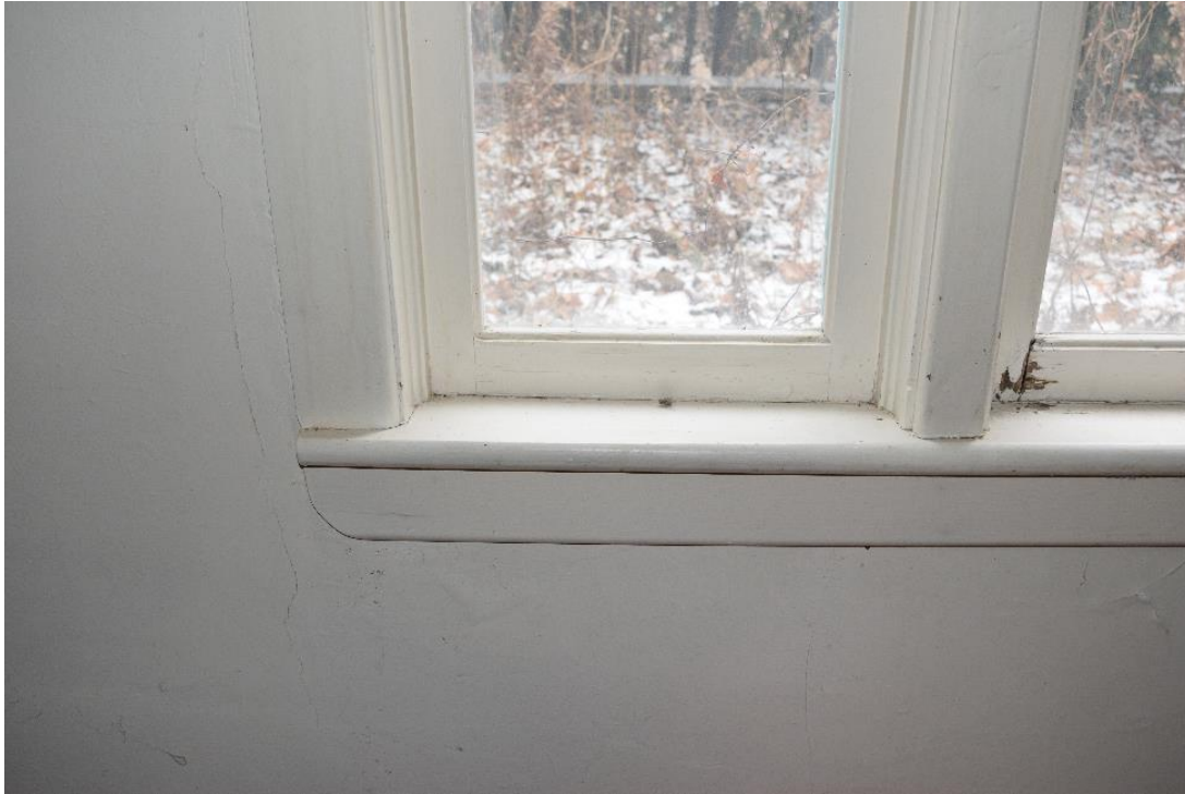
Image 40: Example of typical replacement window trim and non original wood windows
