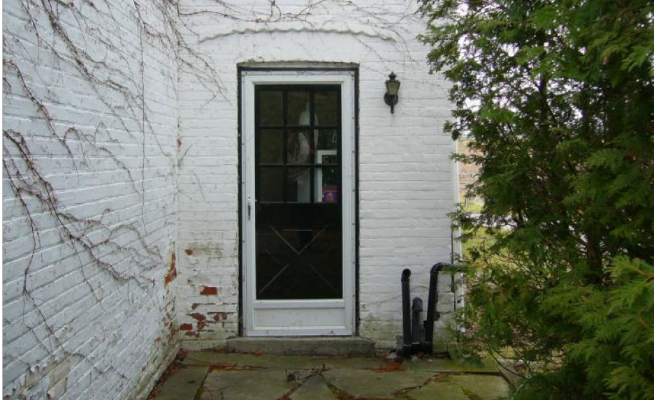
Image 16: Side entrance on east elevation, note recent interior door and storm with original hood moulding
