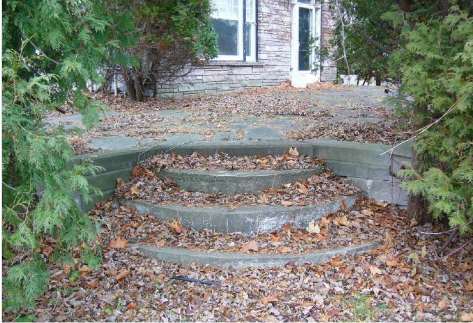
Image 14: Cast concrete steps leading to masonry patio.
