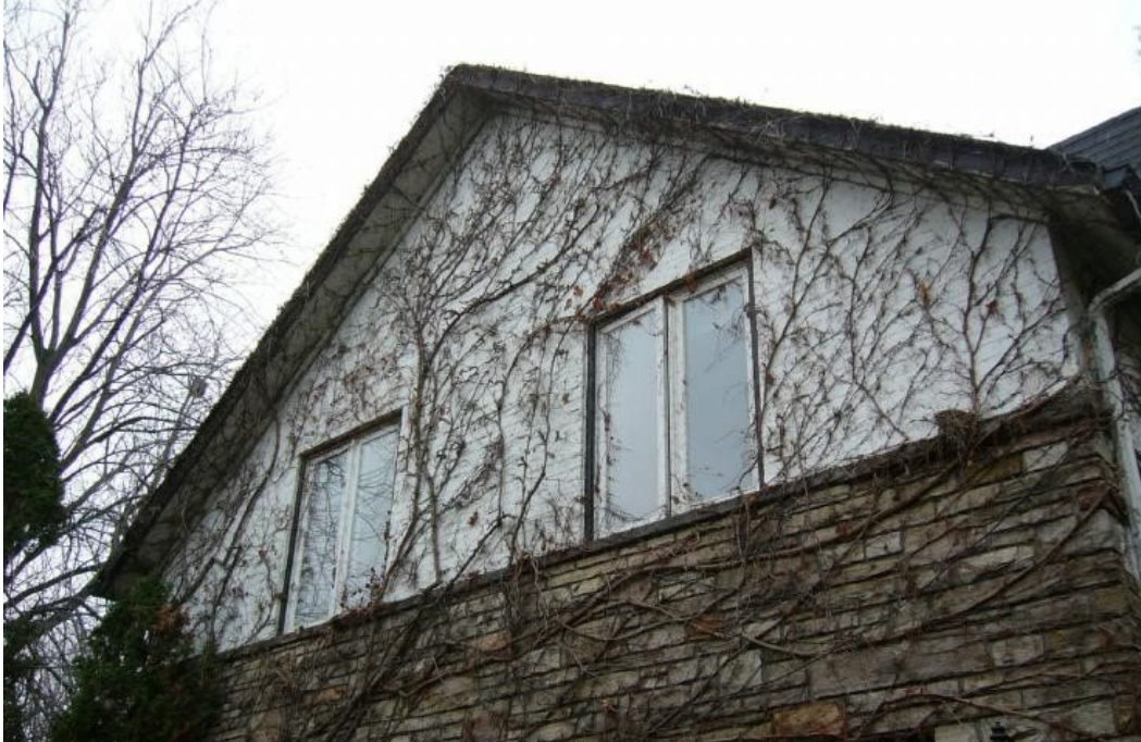
Image 12: modern casement windows on upper storey with painted brick
