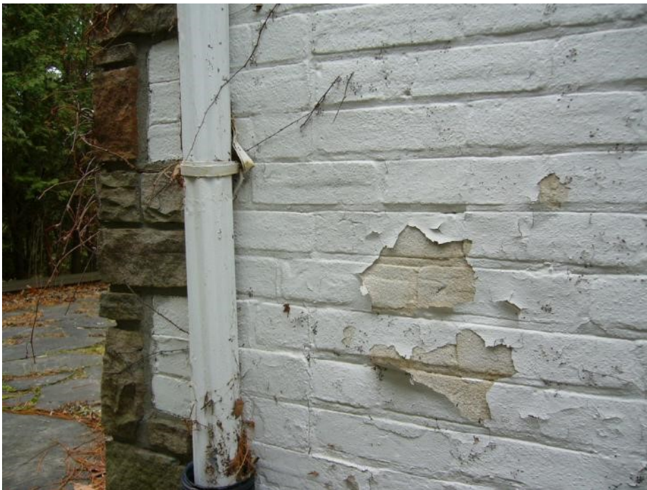
Image 15: Applied stone finish over painted brick wall
