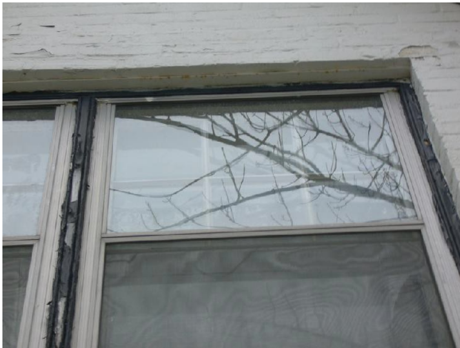
Image 29: Steel lintels support brick courses above. Windows and aluminum storms are not original.
