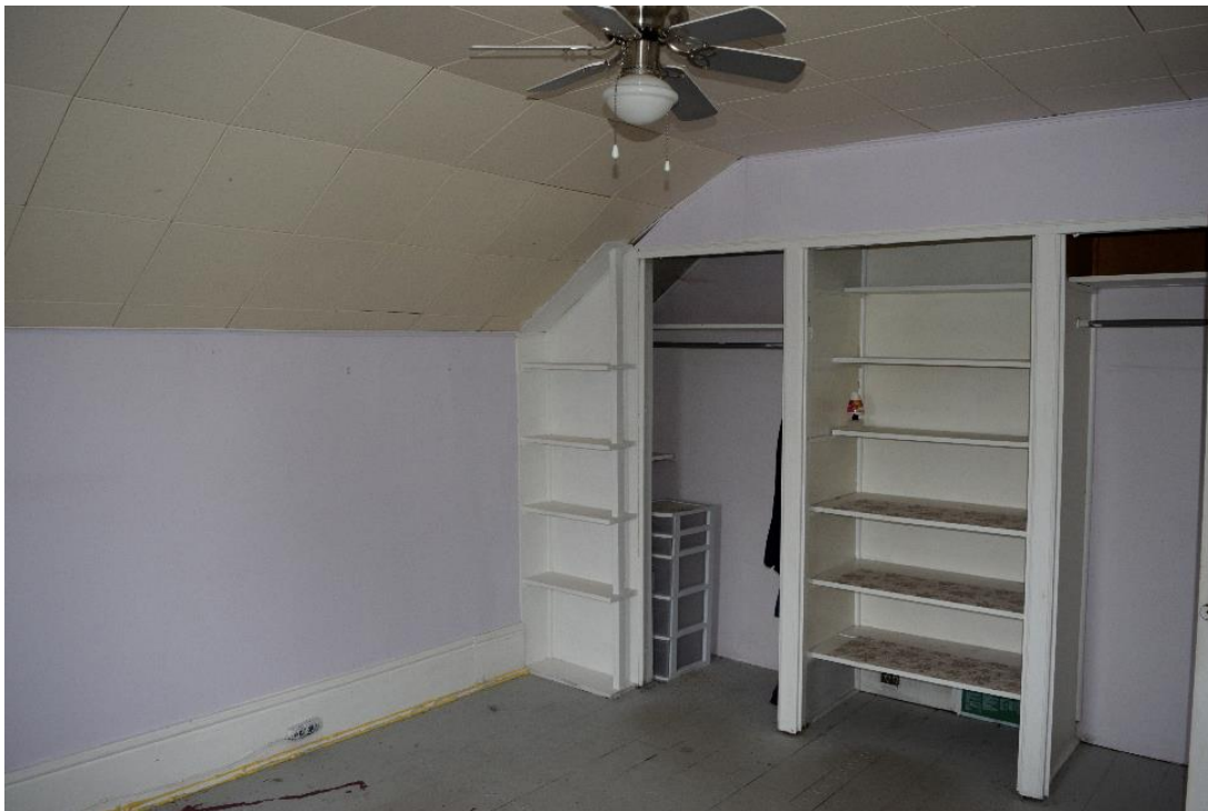
Image 41: Northeast bedroom second floor, note original plank floors and original baseboard, ceiling has been replaced with acoustic tiles
