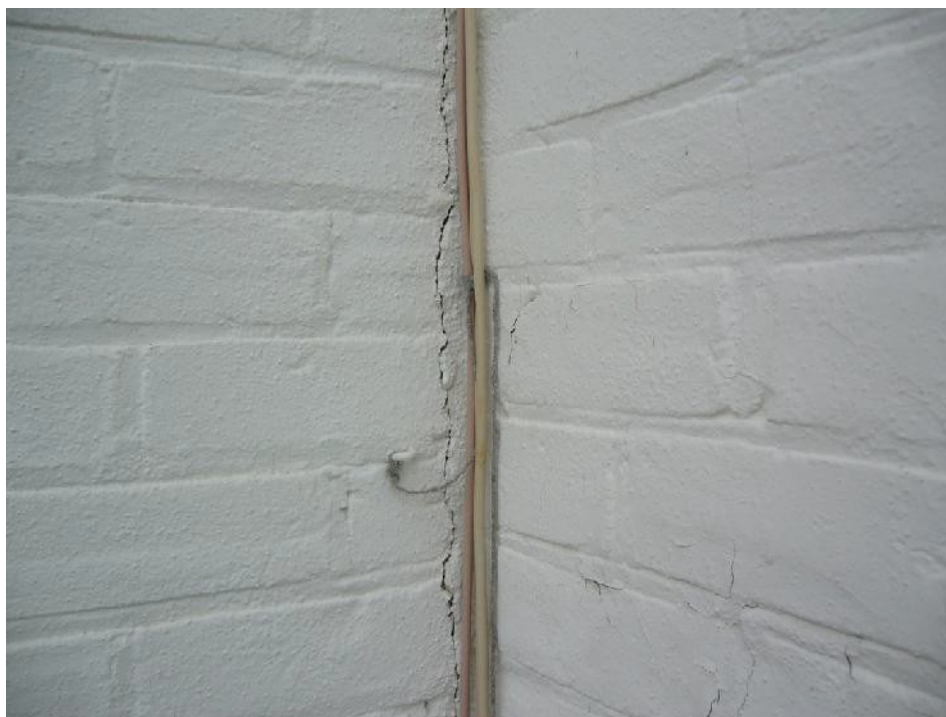
Image 33: Close up of the junction between building masses showing misalignment of brick courses
