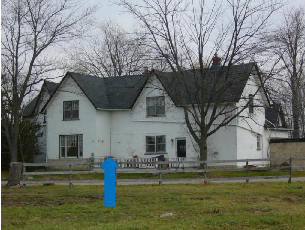
Image 28: North face, blue arrow indicates junction between original construction and later addition
