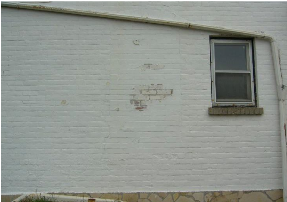
Image 26: The lower floor window under the upper floor window has been blocked up and a new window inserted to the right. The lower brick courses have been covered in masonry cladding.
