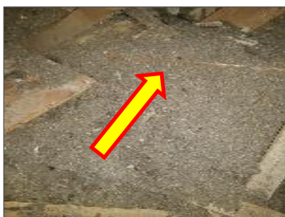
Non-asbestos blown-in attic insulation.
