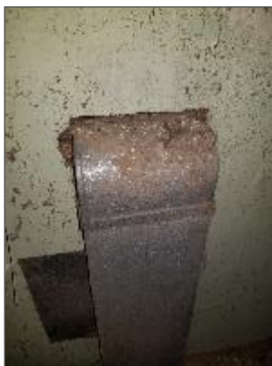
Uninsulated duct, Attic space.
