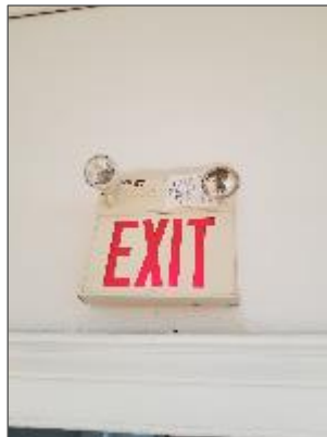
Emergency lighting with lead-containing batteries, Front Entrance Vestibule.
