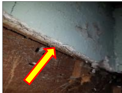
Non-asbestos plaster on wall, Attic space.
