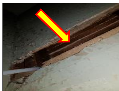
Non-asbestos mortar, Attic space.
